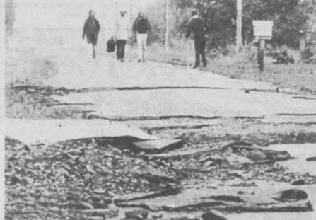
● Three Twyford Rd farmers returned to their properties this morning along a flood-damaged road. Water had ripped up tarseal roads and damaged a bridge.
