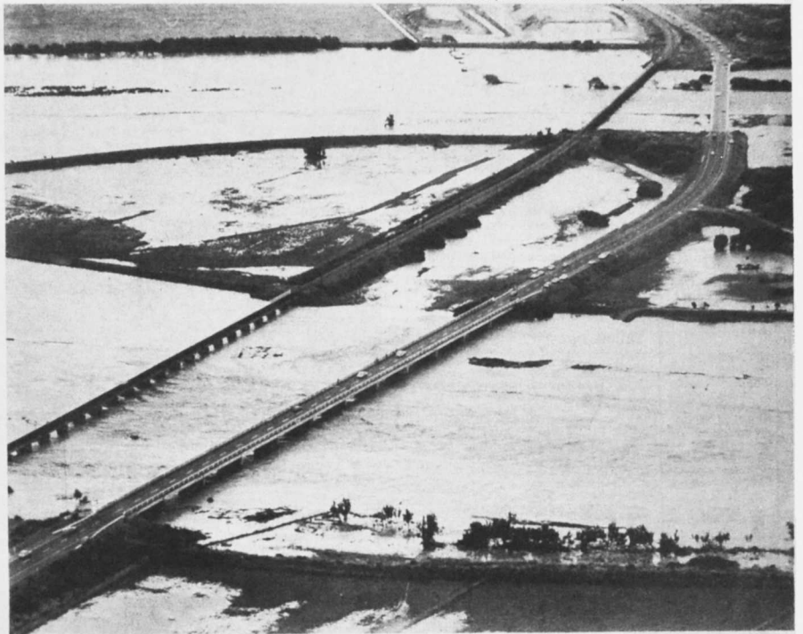
● This was the scene at 11am yesterday as the swollen Ngaruroro and Tutaeuri Rivers passed under the rail and road bridges at Waitangi. The flooded rivers merged into one to punch a big opening into the sea.
