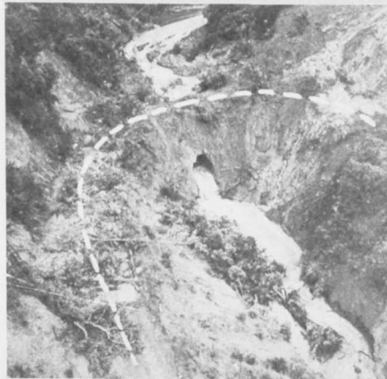
● Above: Heavy rain during the Christmas period created havoc on sloping high country in Mangletton, causing debris to fall from hillsides on to the Mangletton Rd across the Tarapeke Gorge. The road's normal path is depicted by a dotted line.
