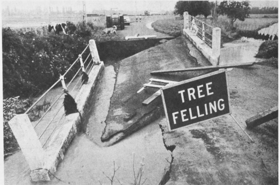
● Floodwater tore a concrete bridge from the road at Twyford yesterday afternoon and the only sign available to warn motorists was for tree felling.
