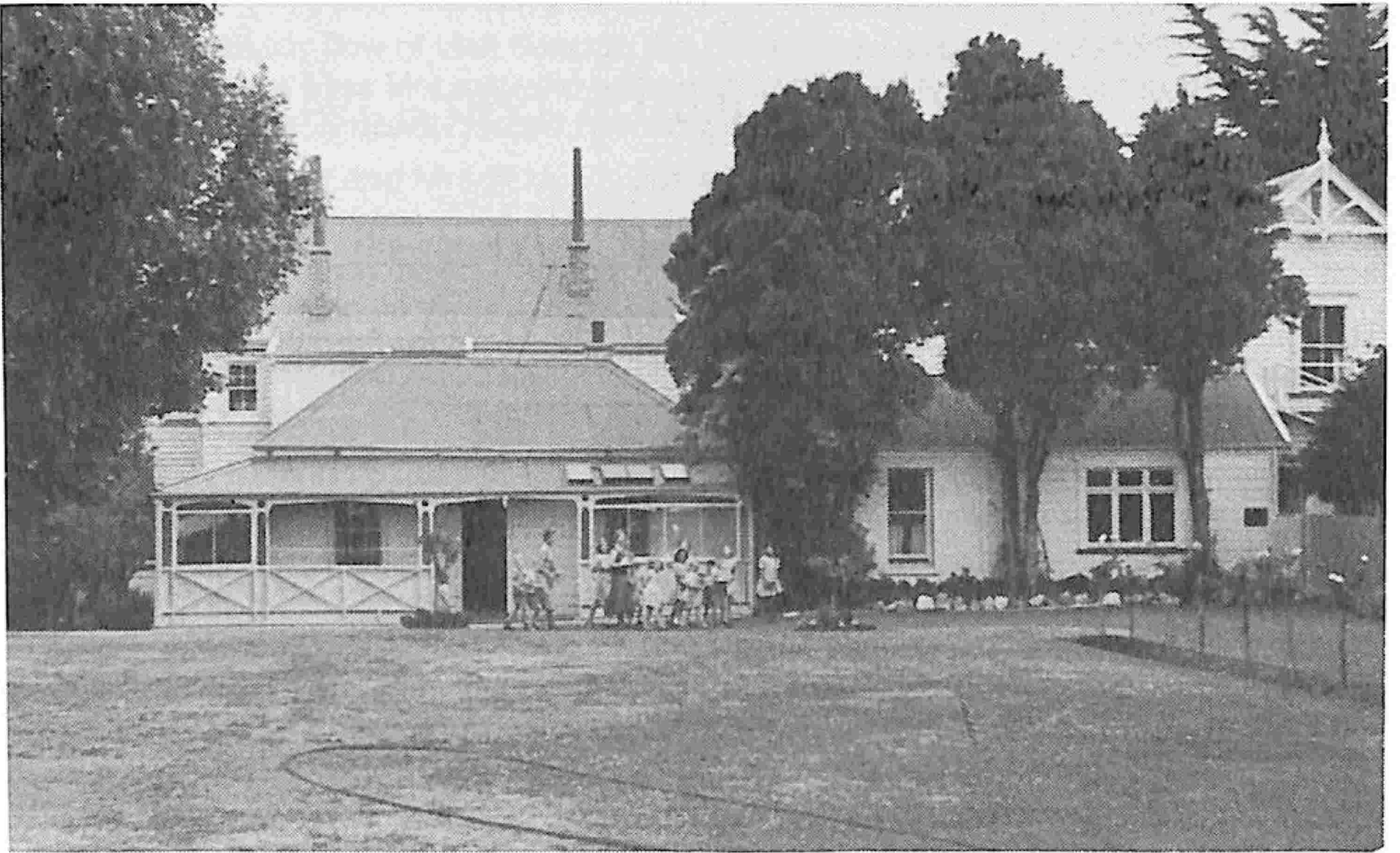
Randall House (Napier Terrace) 1955.
