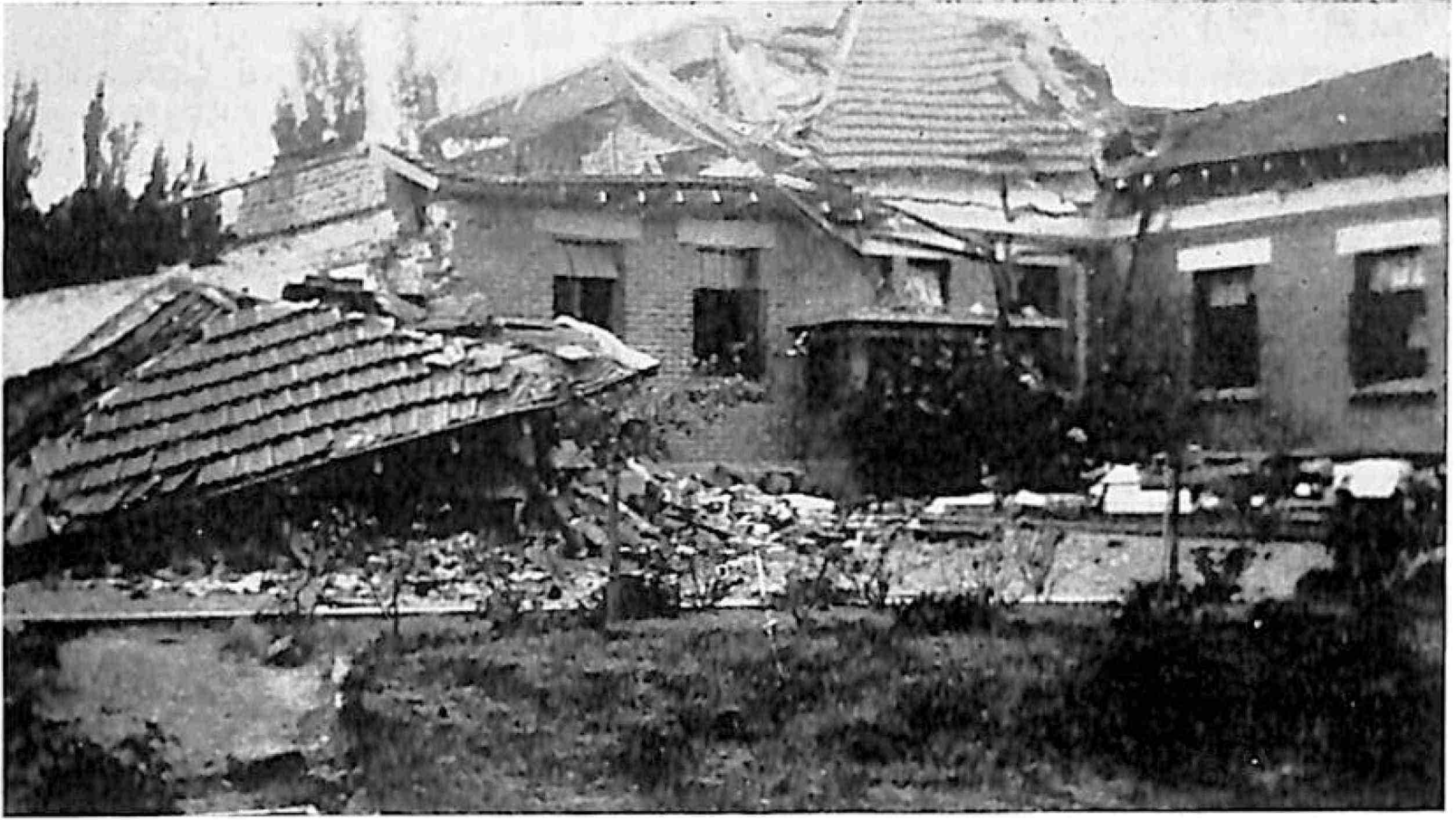
ORIGINAL FRANCE HOUSE AFTER EARTHQUAKE—1931.
