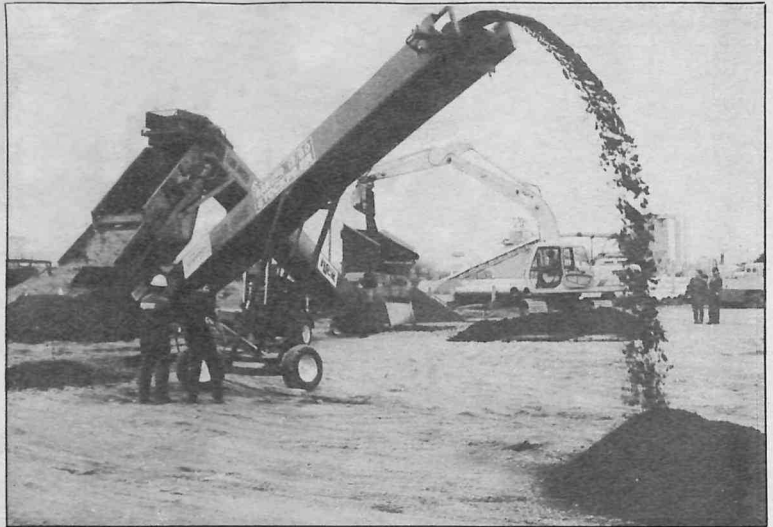
Tuck Contractor's new mobile screening plant.
