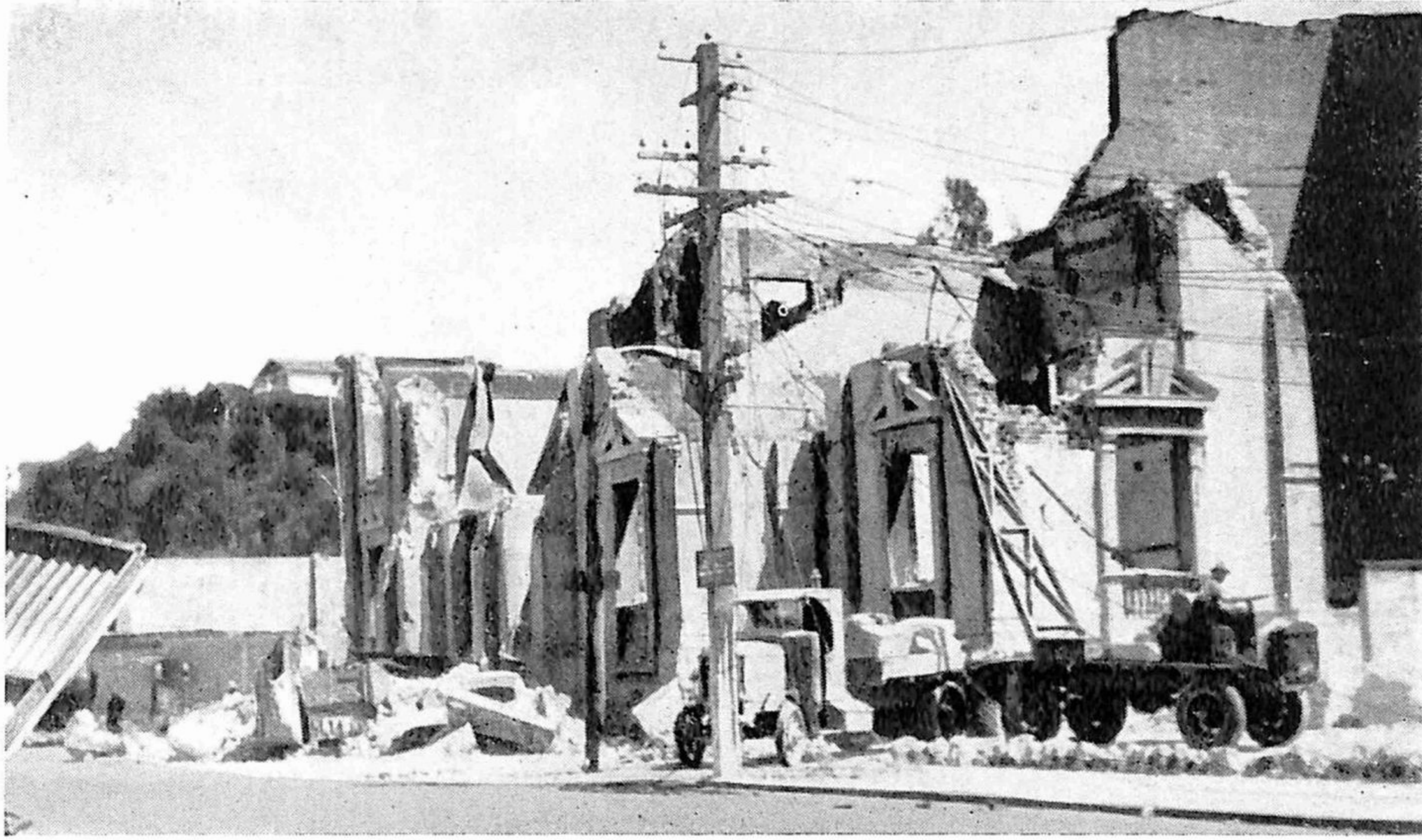
● CLEARING THE DEBRIS—AFTER THE DISASTROUS EARTHQUAKE OF 1931.
