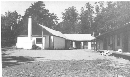
The "Ormatua" Guide Complex, 1986.
