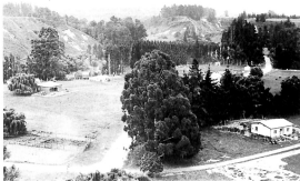
Rissington Valley from top of "The Cutting" — circa 1920
