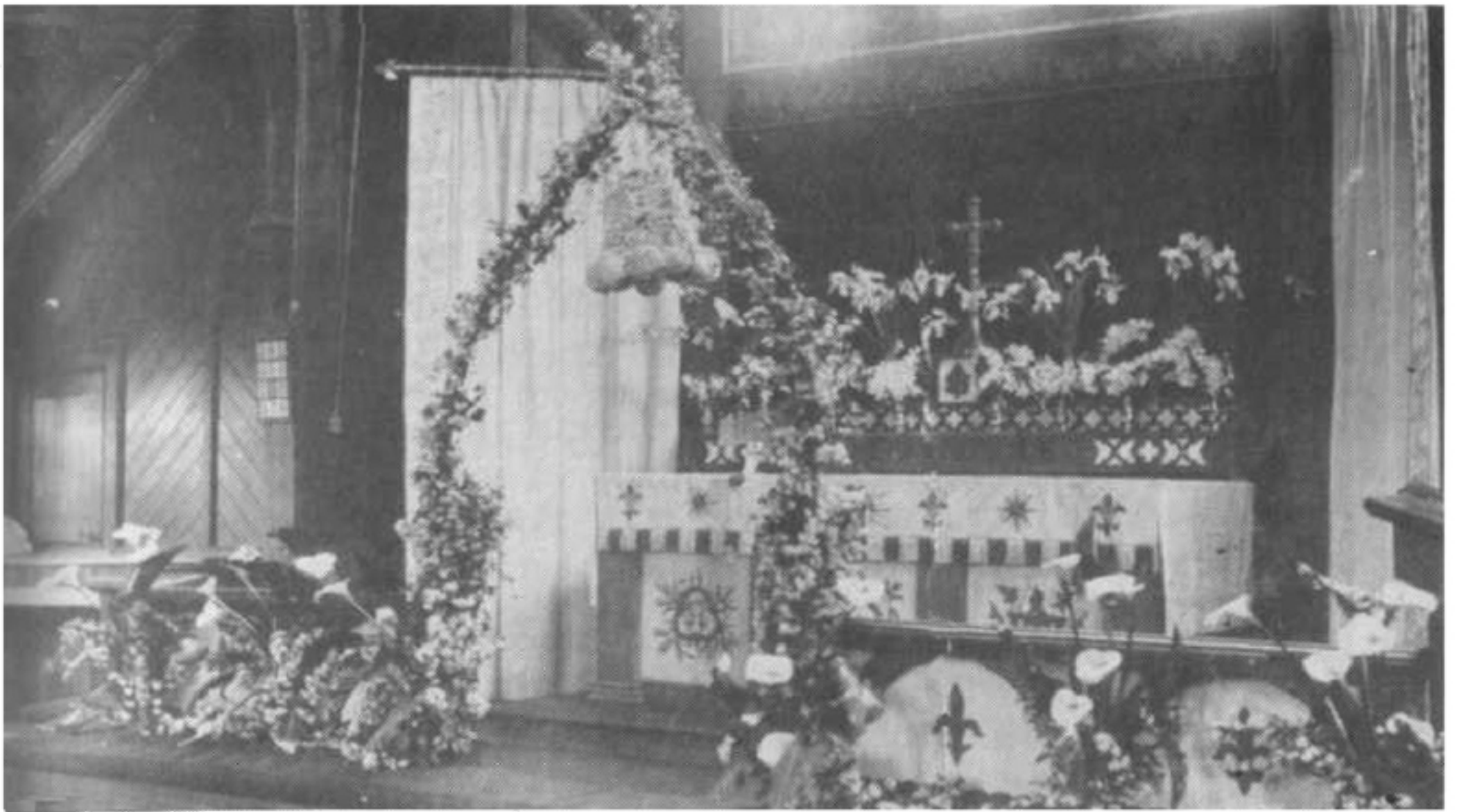
Internal view of 'Mountfort' church before extensions built
