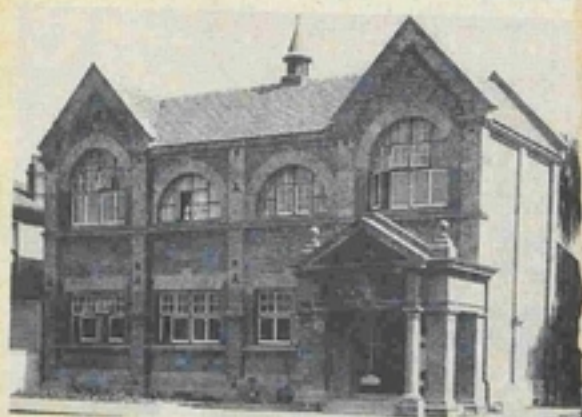
The Hastings Carnegie Library, a brick building with no reinforcing.
