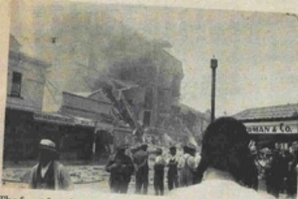
The front façade of the Grand Hotel fell away immediately after the 1931 Hawke's Bay Earthquake.
