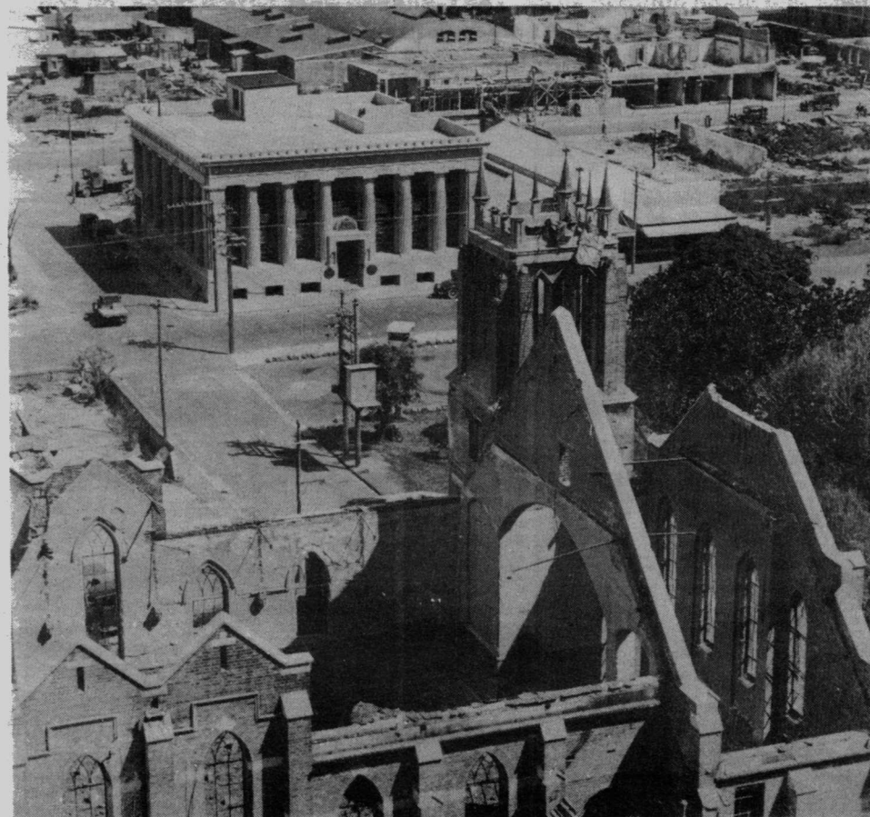
ST PAUL'S CHURCH, Tennyson Street, (foreground) which, nearing completion, withstood the earthquake only to be destroyed by fire. Opposite is the Public Trust Office which was one of few central city buildings to survive.
