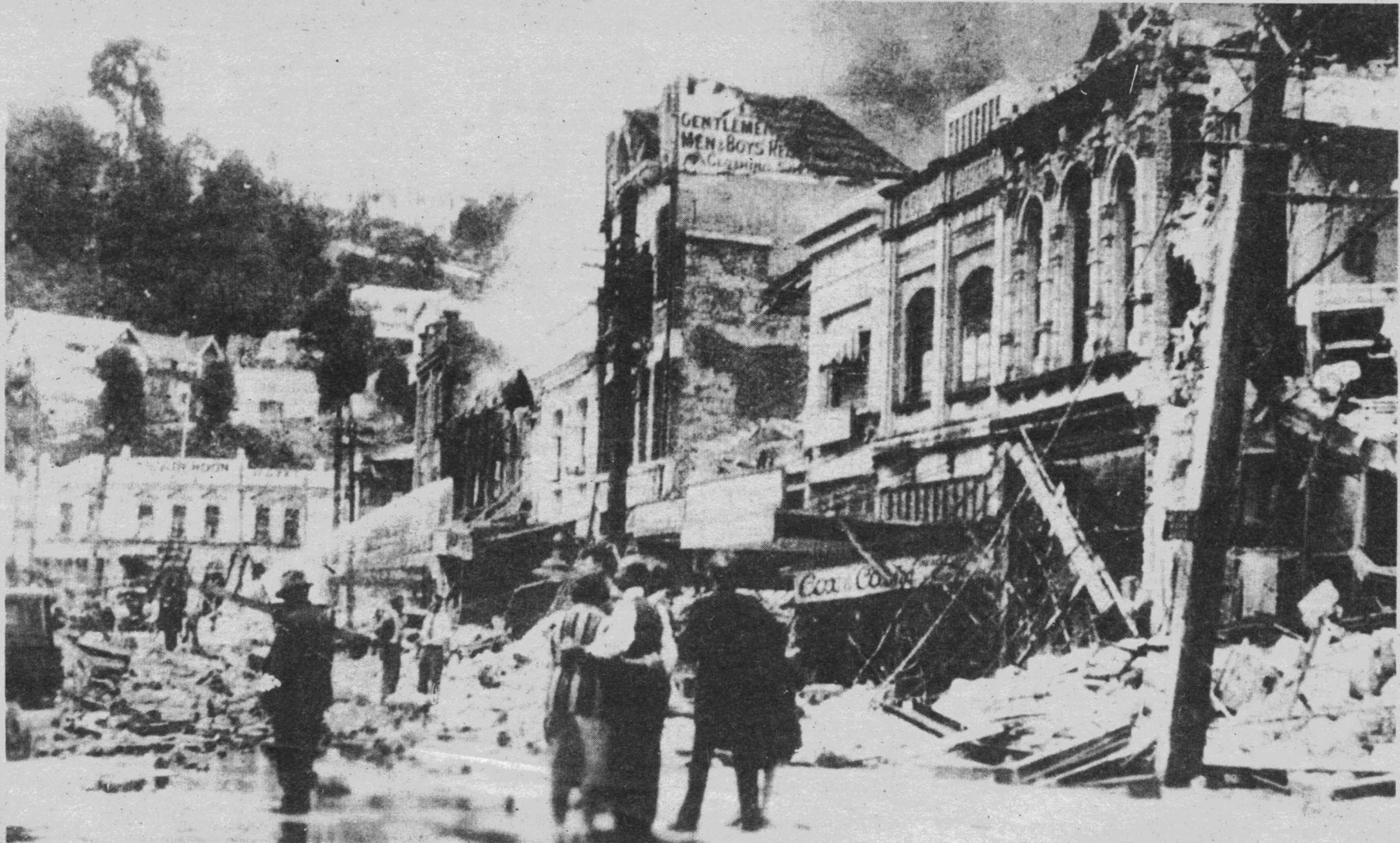
DESTRUCTION in Hastings Street, looking towards Shakespeare Road, Napier.
