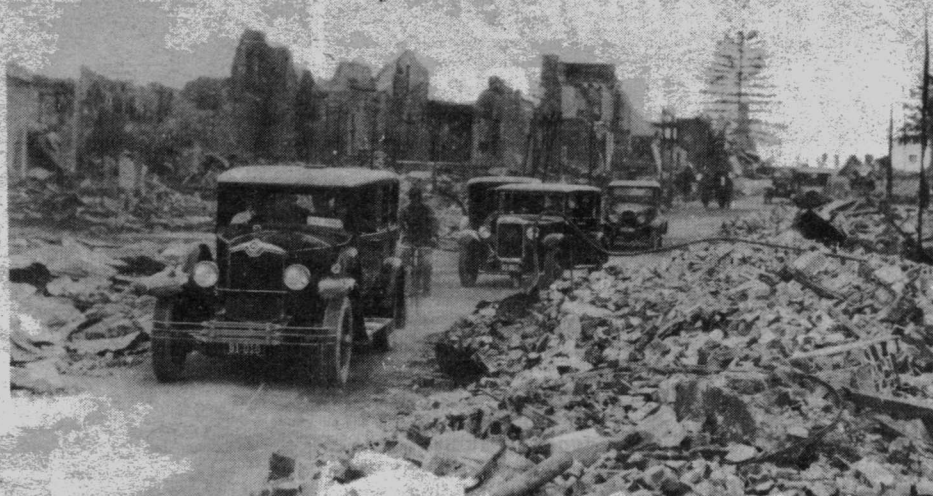
EMERSON STREET — looking towards the Marine Parade — after the earthquake with little room for traffic to work its way through the rubble.
