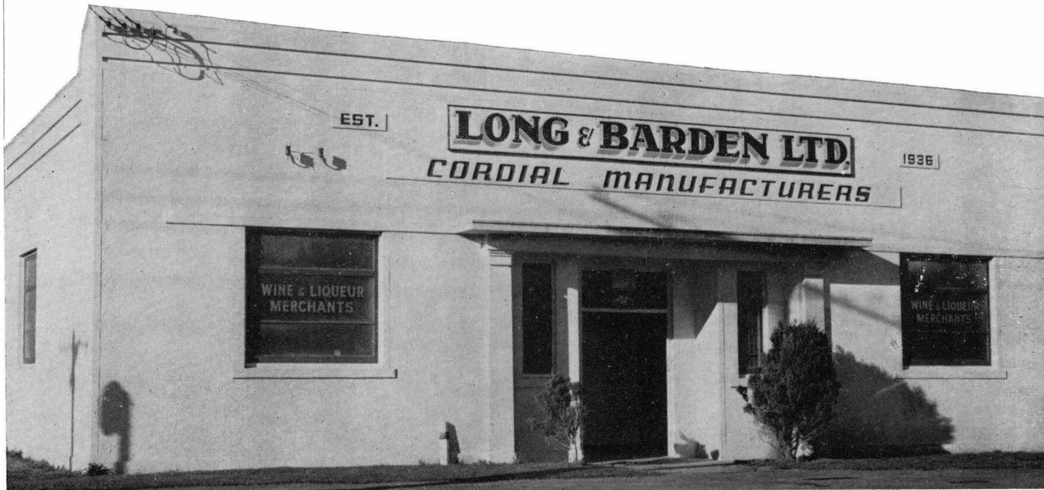
The recently acquired premises of Messrs. Long & Barden Ltd. in Heretaunga Street, Hastings
