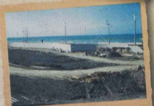
The Sunken Garden taking shape.
