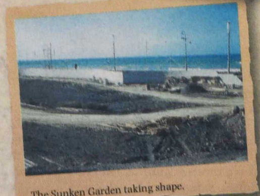
The Sunken Garden taking shape.
