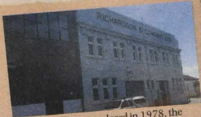
Though the business closed in 1978, the name Richardson & Company still adorns its old building in Ahuriri.
