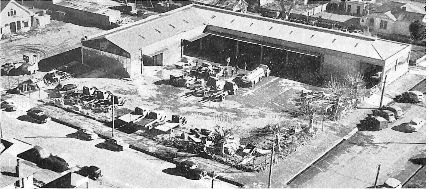
Present Baillie Motors Bedford Trucks Division and Engineering Shop. This central three-quarter acre block, corner of Queen and Nelson Streets is the site on which it is proposed to build modern premises to become Baillie Motors Headquarters.
