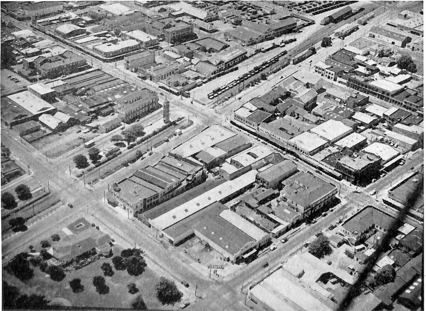
A recent aerial view showing part of the business area of Hastings. The town covers an area of 2,613 acres, of which 130 acres are occupied by well-planned parks and reserves.
