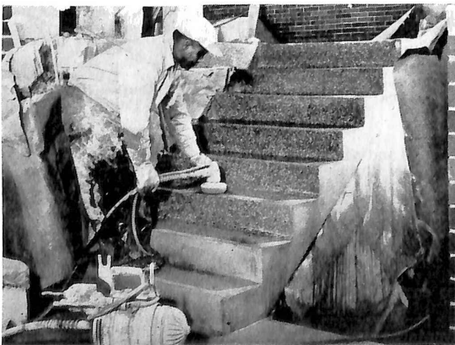
Applying a film of "Surco" to a terrazzo surface.
