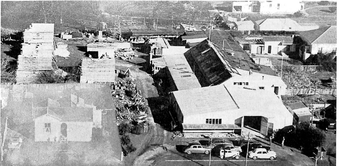
An aerial view of the factory and yards
