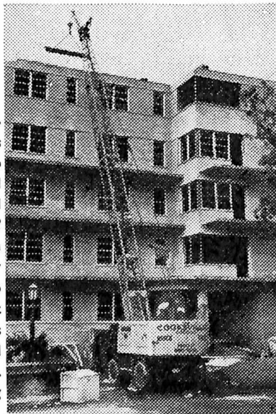
A Coles with 60' jib and 12' fly jib handles building components for a block of flats in Canada . . .
