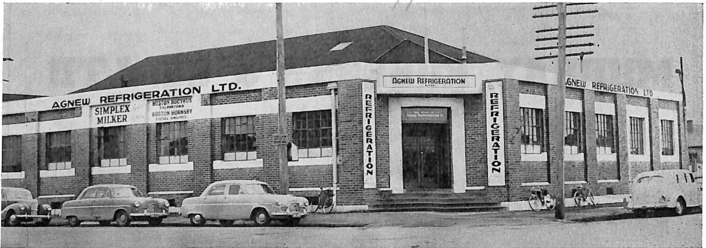
The firm's head office in Karamu Road, Hastings, incorporates showrooms, offices, bulk stores, service departments and an engineering department.
