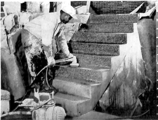
Applying a film of "Surco" to a terrazo surface.
