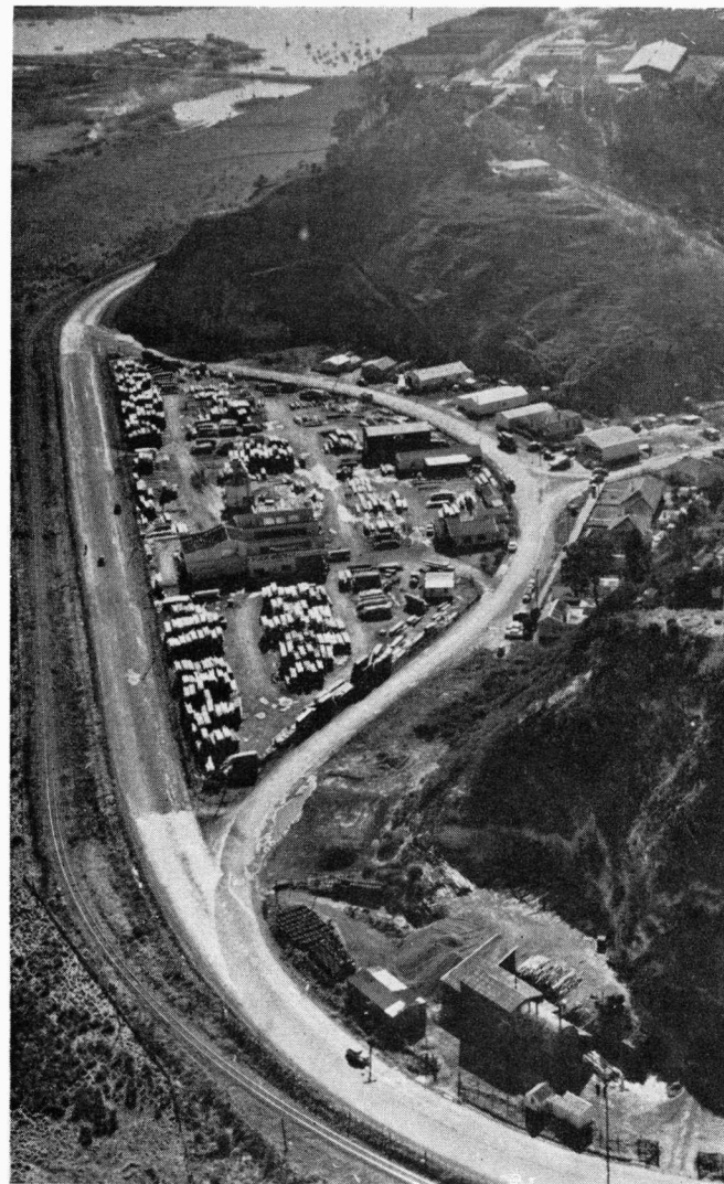
● A modern timber mill stands here at Conunna Bay where once the early trading vessels anchored.
