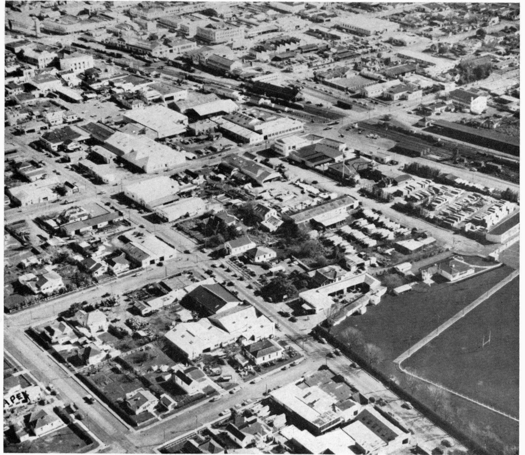
● Many industries are centred around Karamu Road North, shown above.
