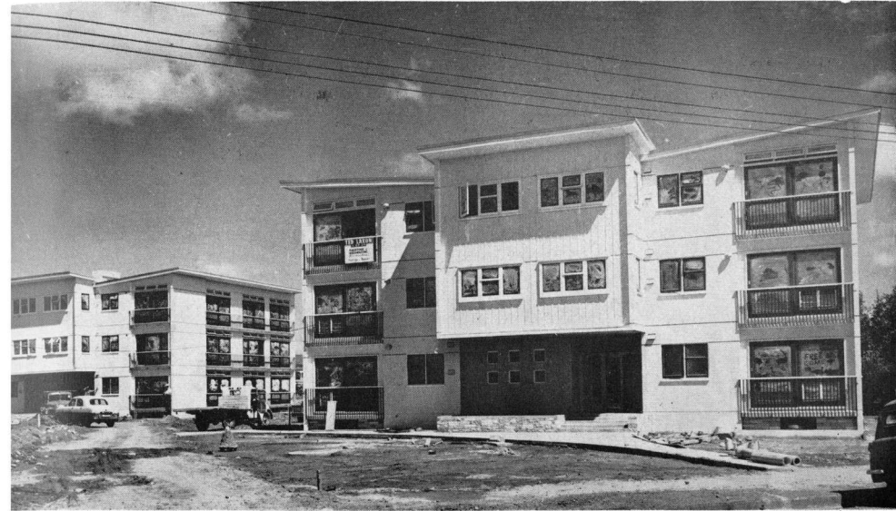
"STAR" FLATS CONTRACT – HASTINGS
