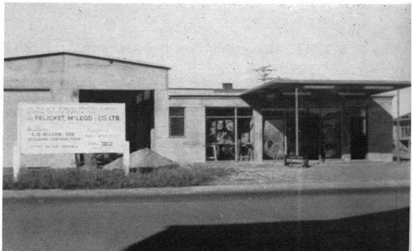
A concrete building.
