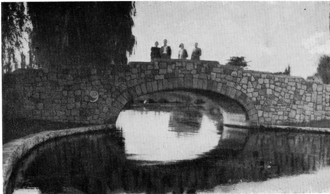
Rustic Bridge, Windsor Park, Hastings
