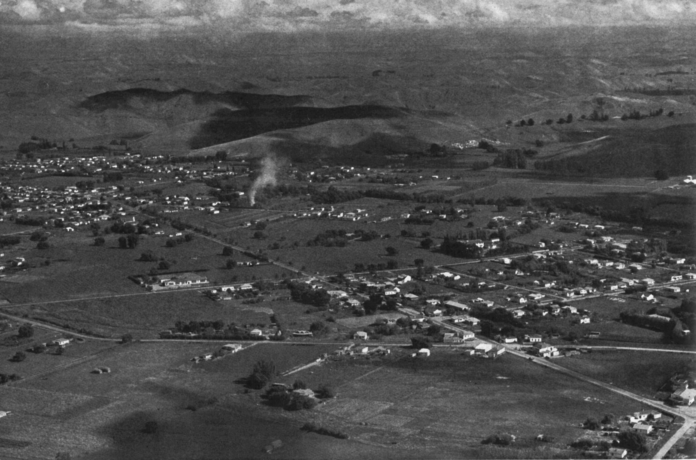
TARADALE (Town District). Pop.: 2630. Area: 1469 acres. 5m. SW of Napier. The neighbouring townships of Greenmeadows and Taradale seen in this photograph are richly productive dairy farming areas towards which the city of Napier is expanding. Situated on flat land but backed by rising hills, there are numerous orchards, some of them established nearly 50 years ago. There are splendid artesian water supplies. The district is noted for the extremely productive vineyards and wine cellars. Very few visitors to the district fail to visit the Hawke's Bay Acclimatisation Society's game farm at Greenmeadows, where several kiwis live in captivity. Pheasants are bred for liberation and hill country provides excellent shooting. There is a Roman Catholic Seminary at Greenmeadows. The district, including nearby Meanee, was established by early military settlers from India.
