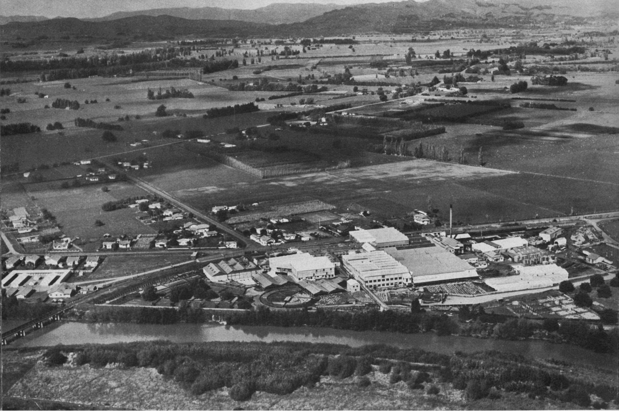
HASTINGS. The countryside shown is typical of the fertile Heretaunga Plain, with Whakatu, one of the two large freezing works in the Hastings district dominating the foreground. Tomoana, the other works, is nearer Hastings, which is in the right distance. These works kill to export over 100,000,000 lbs. annually and during the season the daily killings in the two works exceed 26,000 lambs. Cattle were formerly grazed on the plains chiefly to break in the pastures, but there is now a large export trade in chilled beef. Some of the world's best pedigree stock has been imported, principally from Great Britain, and the prime condition of the 74,000 carcasses now passing through the two meatworks each season has meant much to the people of Britain. The river in the foreground is the Ngaruroro. It flows into the sea near the settlement of Clive, which is on the road midway between Hastings and Napier.
