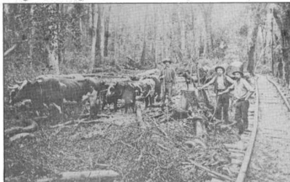
From Takapau to Woodville, wooden tramlines snaked into the bush. Logs were brought out on the tramline to the sawmills and the railway line.
