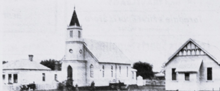
THE old St Columba's Church on its Gloucester Street site, flanked by its social hall, built in 1916, and manse.
