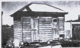
ANOTHER tiny building from the early days, but one with a rather different use — Taradale's first lock-up.
