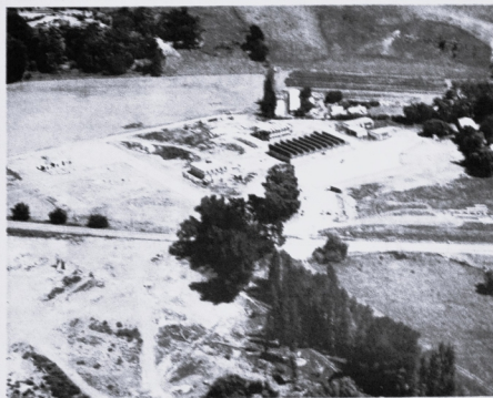
THE Hawke's Bay Community College under construction at the end of 1974. It opened to its first classes of apprentices the following year.
