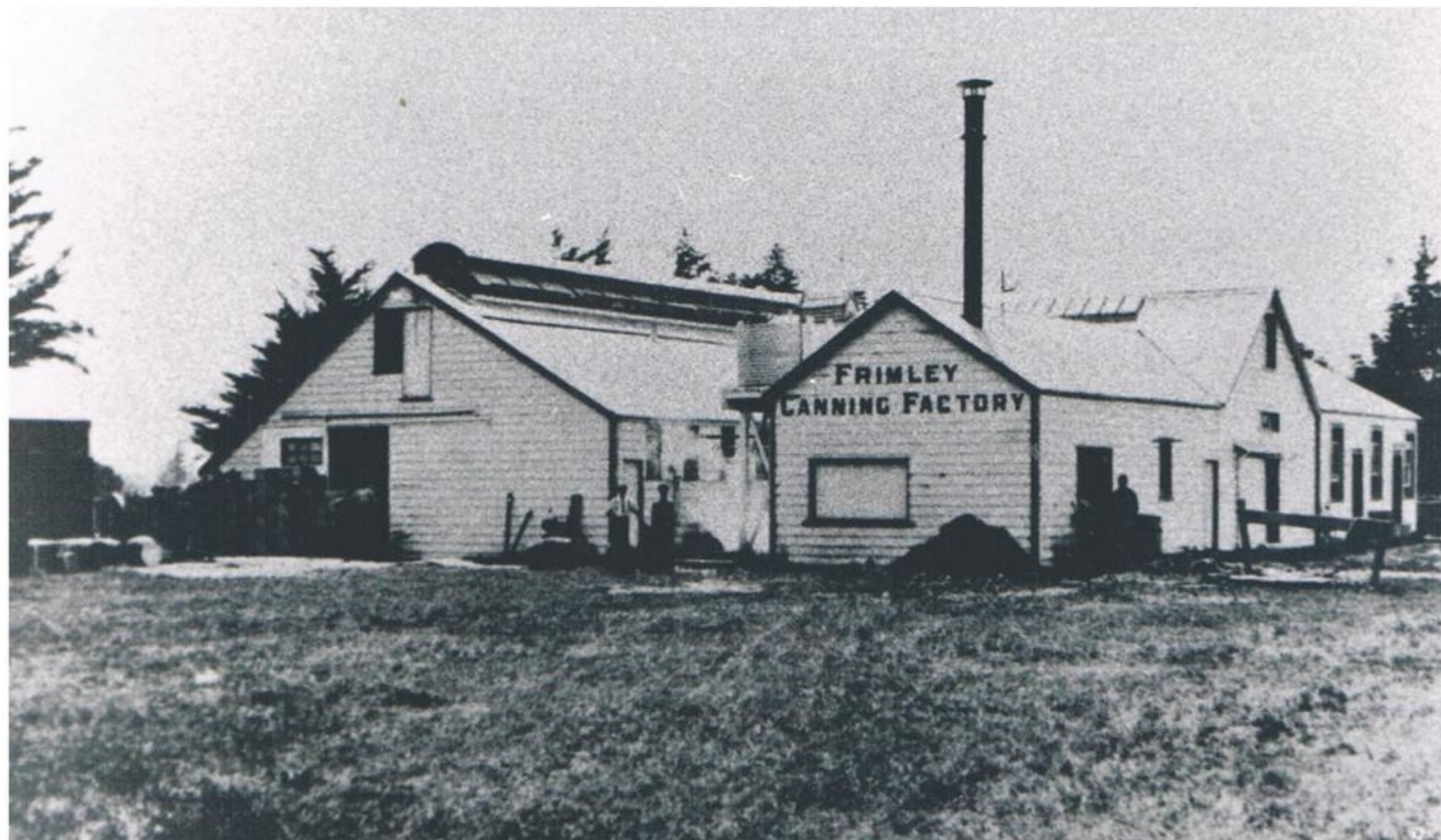
Early View. The factory growing from the converted woolshed
