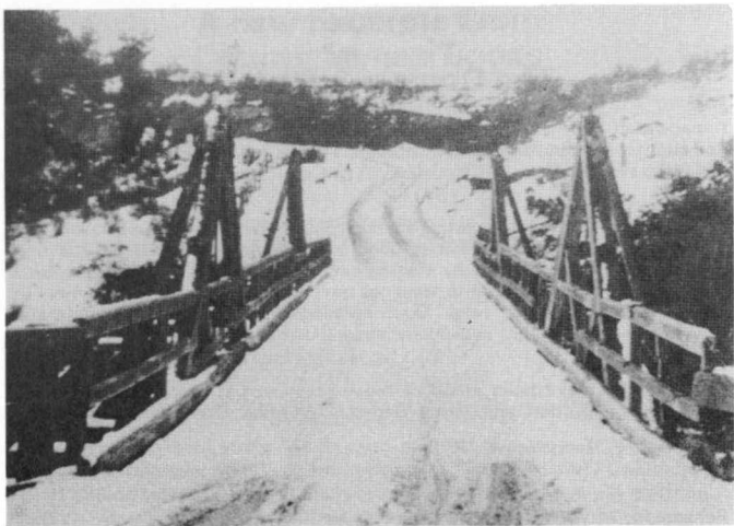
Road bridge over Makotuku Stream in winter.
