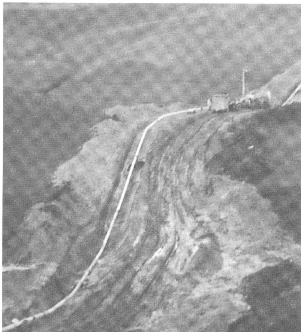
Lying of gas pipeline through John Gray's
