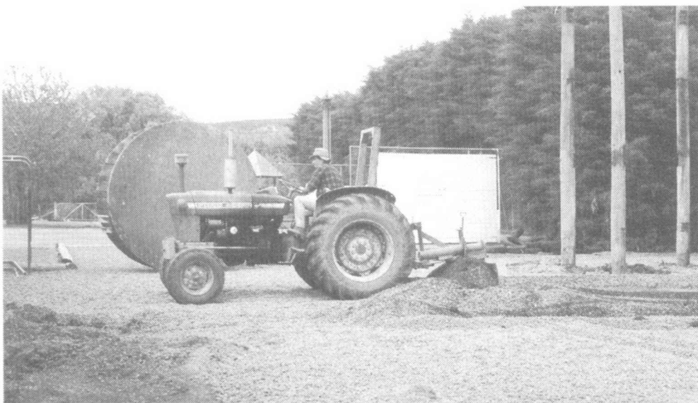
Demolishing old adventure playground 1996 (Margaretha Butler)
