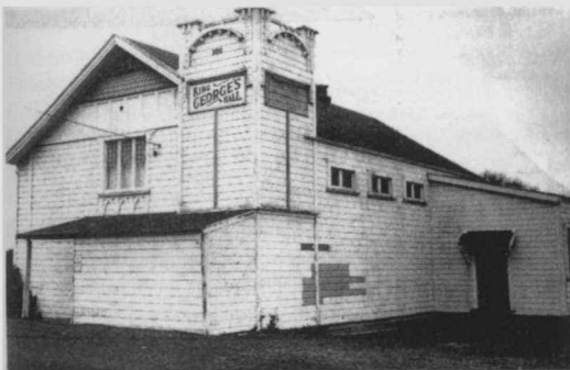
A derelict King George's Hall.
