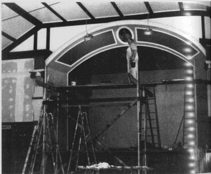
Herbert (Herbie) Kempton painting the timber mouldings on the curved arch of the proscenium, 1988. He has completed the rosettes and has started on the pilasters each side of the stage.
