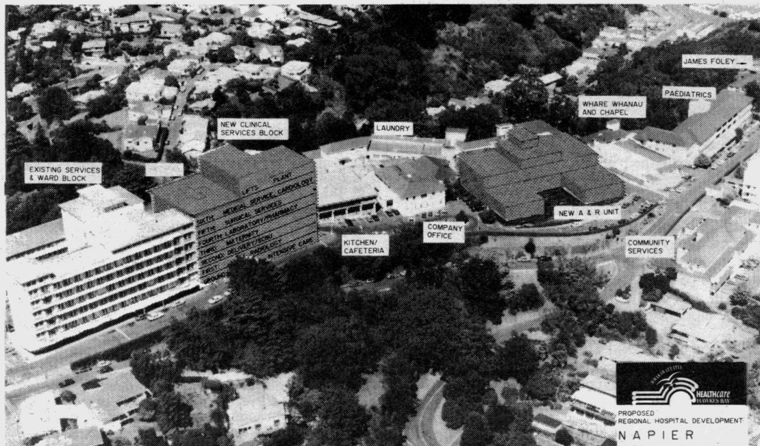
The design for a Regional Hospital for Napier that was considered by the Task Force. It shows a new seven storey clinical block and a new Assessment and Rehabilitation Unit.
