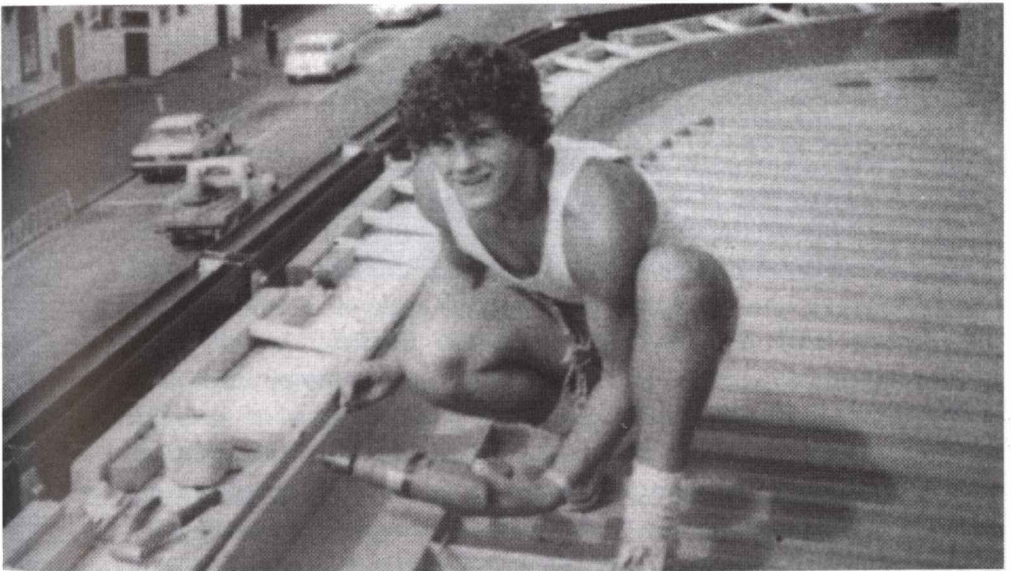
Aaron Gardner a trainee at the Ruahapia Construction Training Unit, on work experience with a roofing contractor. Tracks training courses included a six week period of work experience during which employers supervised trainees and provided extra training.
