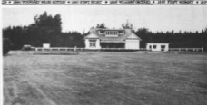
The Hastings Golf Club's 80th house, at Bridge Pa, is getting an established look. In 1912, the area was a barren thicket where E. J. Watt built the clubhouse. In the ensuing years, the clubhouse additions in the centre were added.
