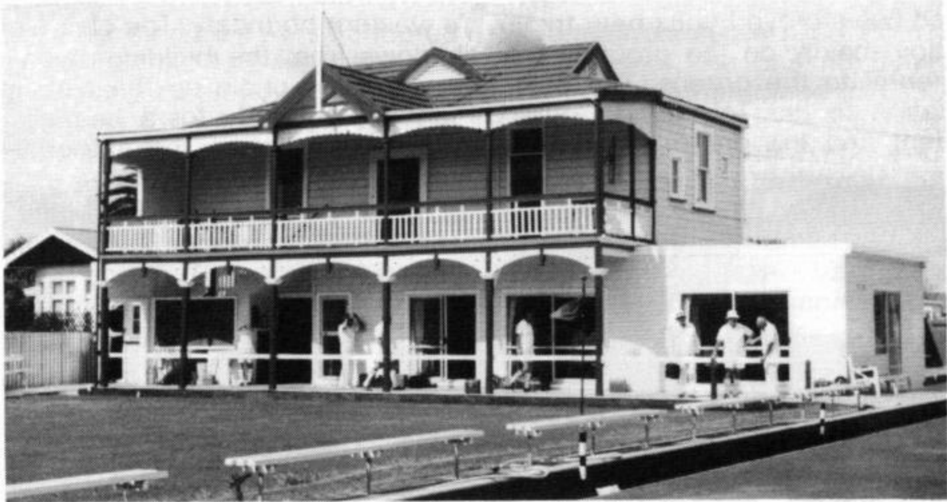
Club rooms after renovations, 1980.
