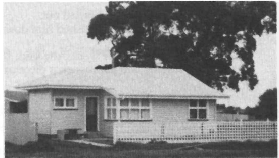
The "flat" now facing Chambers Street.
