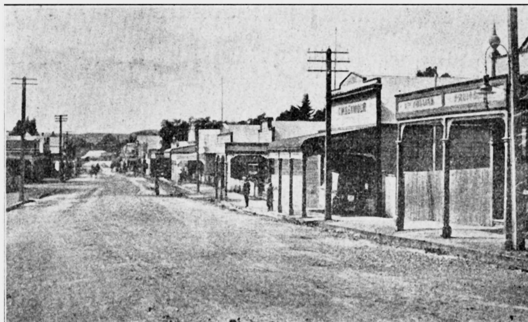
1908.—RUATANIWHA STREET, LOOKING EAST, TAKEN FROM A POINT WHERE McLEAN'S GARAGE NOW STANDS. THE RIGHT CORNER IS THE PRESENT LOCATION OF THE MUNICIPAL THEATRE.
