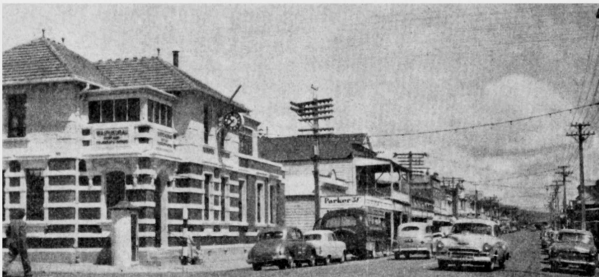
PRESENT DAY VIEW OF RUATANIWHA STREET, LOOKING WEST FROM THE POST OFFICE.
