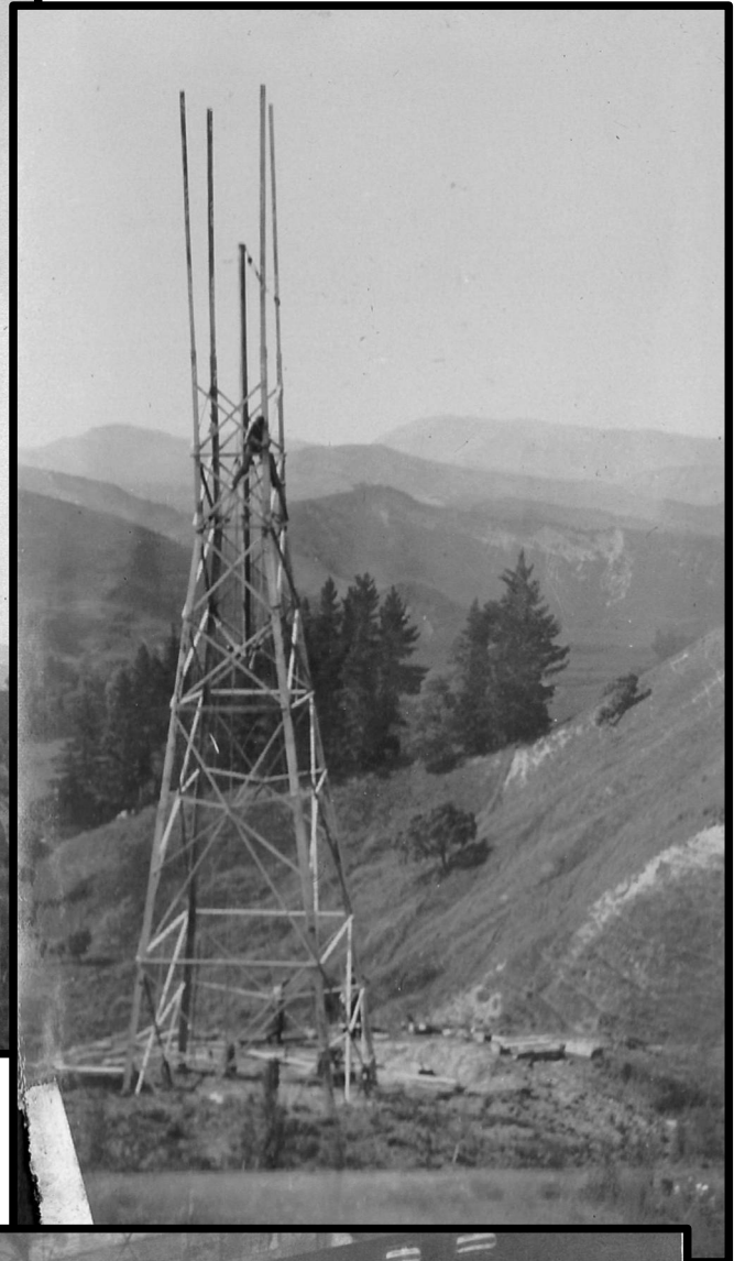
Building an angle head at Waihi
