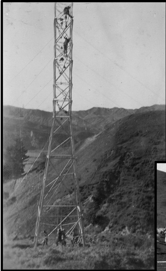
Hanging wire on an angle head tower 260
