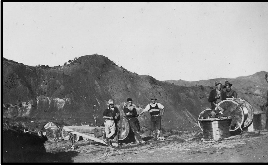
Cable mounted, ready for running out
