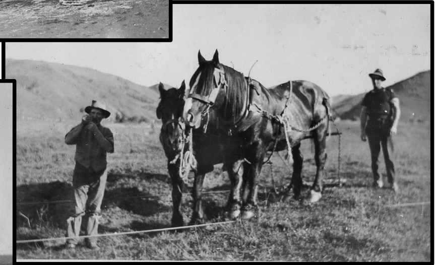
Motive power for running out cables
