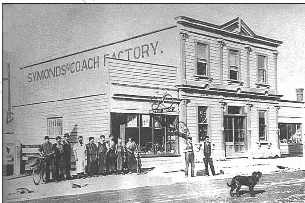
The two building fronts for William J. Symonds Coach Factory and his adjoining Cycle Depot on Queen St east, these buildings burnt down January 1906
