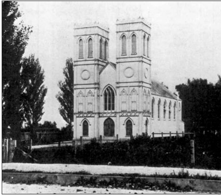
St. Matthew's first wooden Church of England with two towers and shingled roof on Section 76 Heretaunga St west at the corner of King St at left edge on land of Mr Vickers and Somerville, opened May 1877 – till 1886, it became a Sunday School and Drill Hall till it burnt down in June 1898
