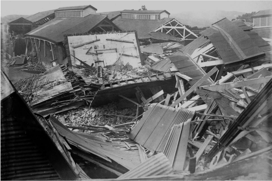
1931, Borthwick Freezing Works damage site with pipes at left, wooden roof ventilation and the Havelock Hills distant, by Sydney Charles Smith
