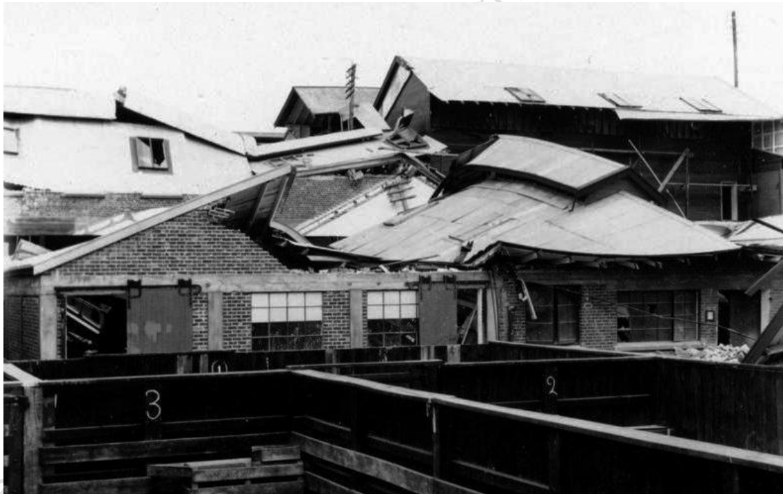
1931, Tomoana Freezing Works earthquake damage
