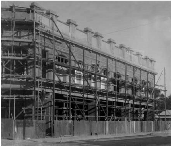
1915, Roach Brothers new mission style ferro-concrete department store being built on the corner of Heretaunga St west and King St where their father originally purchased the business from T. A. Hayes in 1884. The two storied brick building designed by Christchurch architect Sydney Lutterell under construction shows Roachs' Drapers Est 1884 and Glasgow House signage corner veranda right edge
