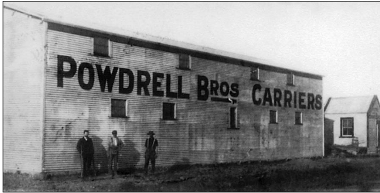
Powdrell Bros, carriers premises on Market St for their traction engine maintenance, a tall shed with two levels of window, poss Barry Bros old stables in Market St and a small entrance office further along
