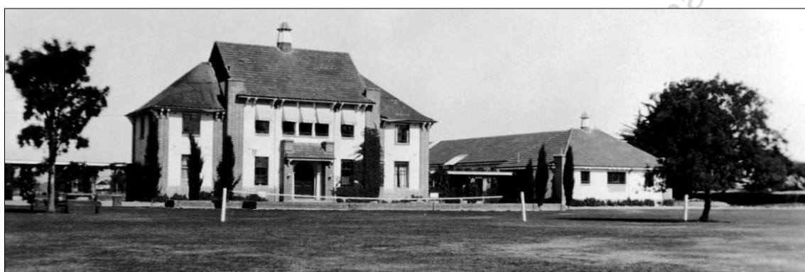
1931 February, Quake repairs to roof
