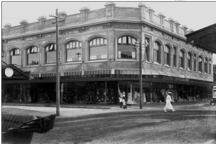
1915 November, Roach's Ltd new mission style ferro-concrete department store opened with plate-glass frontage of 100 feet on the corner of Heretaunga St west and King St opened taken 1920c from the side of the Cosy De Luxe Theatre, by Stefano Webb. This store collapsed in the 1931 earthquake with 17 fatalities.
