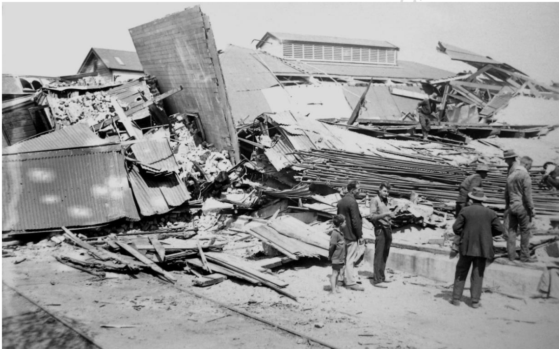
1931, Borthwick Freezing Works near railway line shows men and boy surveying the damage with pile of pipes spread behind note vertical wall with window below, wooden roof ventilation, by Sydney Charles Smith
