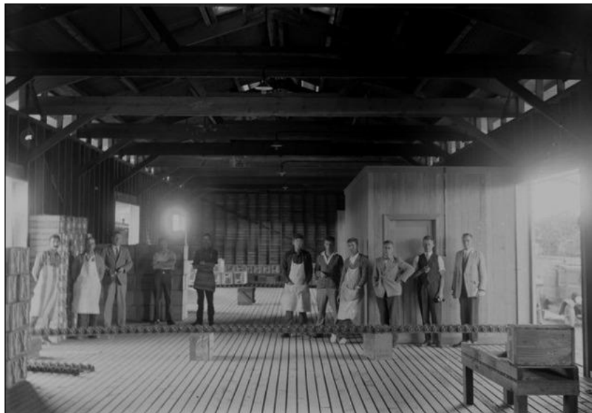
1930's, looking north shows a group of workmen posing inside the narrow fruit grading shed (some in suit jackets and some in aprons) at the Hawke's Bay Fruitgrowers' Federation siding on Karamu Rd sth. Wooden fruit crates and conveyor rollers for loading crates on to rail wagons and old ford truck through doorway on right, by Henry Norford Whitehead
