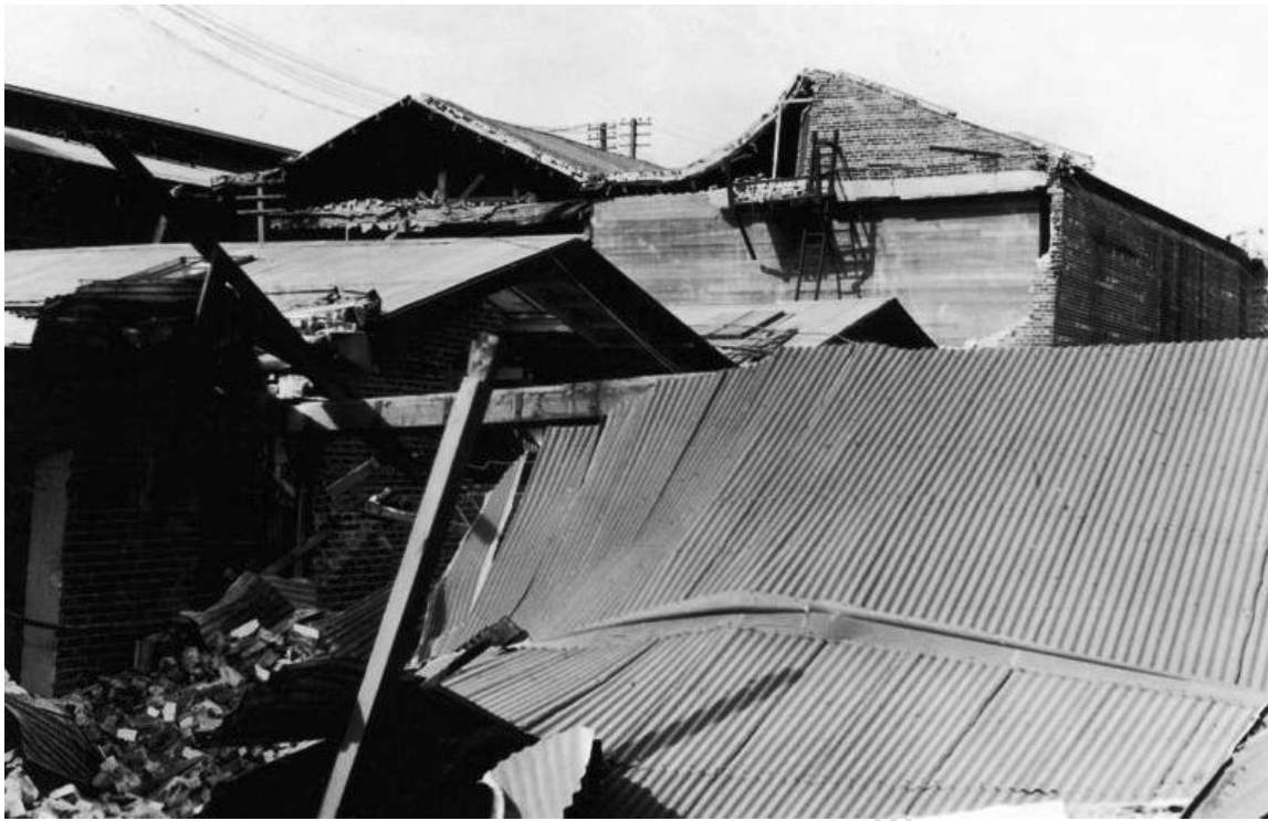
1931, Tomoana Freezing Works earthquake damage
