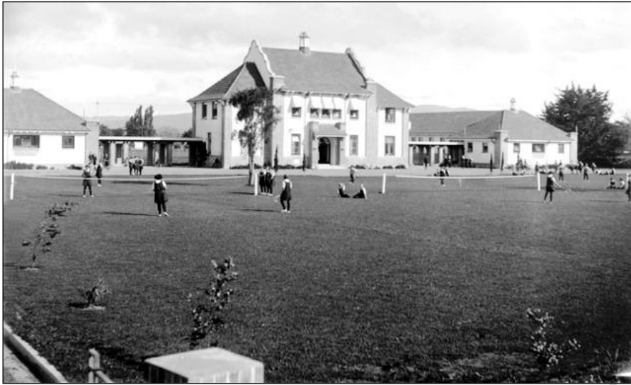
1920's, The Hastings High School taken from the gate shows the Main building of a Cape Dutch design with Doric pillars, the east wing and west wings, girls playing tennis and sapling trees planted and the extended Karamu Rd sth
