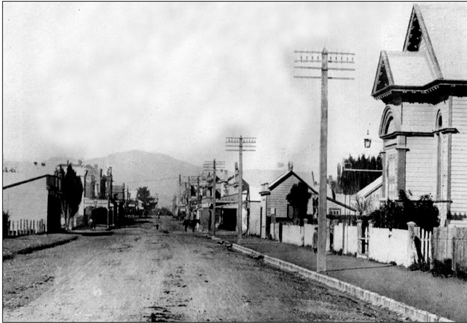
Heretaunga St west looking east from Nelson St taken aprox 1905 with telegraph poles, shows a building without veranda near right, then G. F. Roach old grocery on corner further up, the trees on left are at King St by the old St. Matthew's Church site and the Art & Pottery Fancy Goods store, Note the large tree growing over the main road in distant near Market St and in photo below
