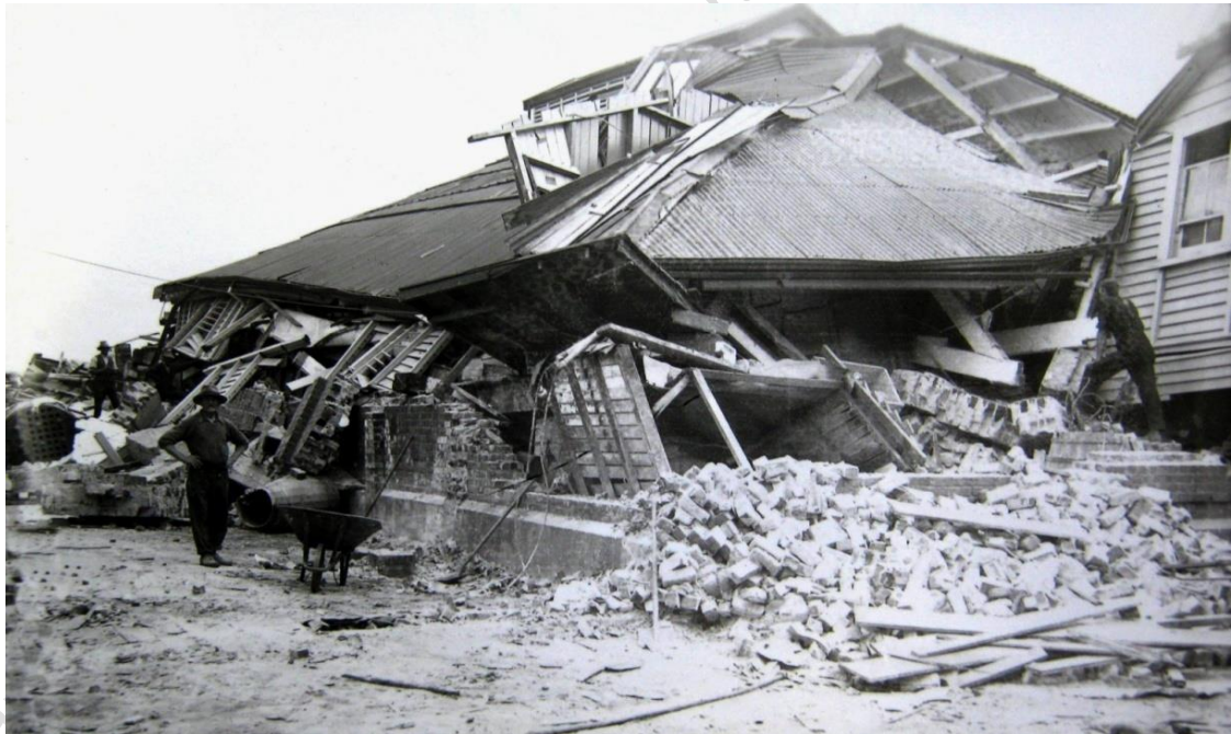
1931, Borthwick Freezing Works shows 3 men working on demolition site with wheelbarrow, wooden roof ventilation, by Sydney Charles Smith
