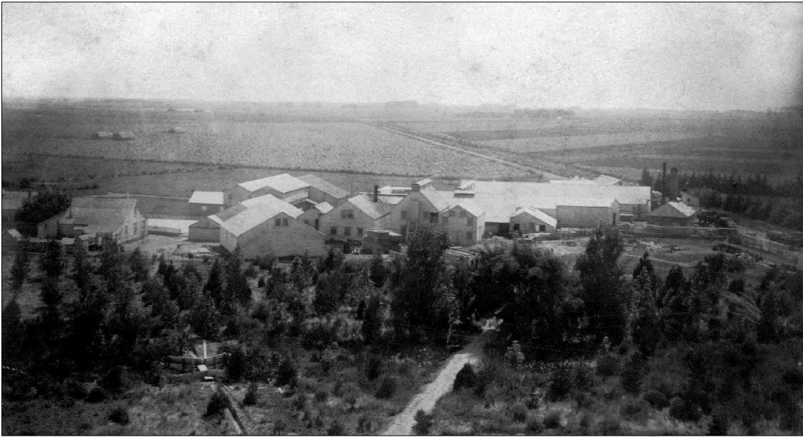
1893, Nelson Brothers Tomoana Freezing Works buildings, shows a cluster of large and small buildings before subsequent fires, mostly tall and narrow with small windows, a tannery, by Andrews Bros of Napier Portrait Studio.
