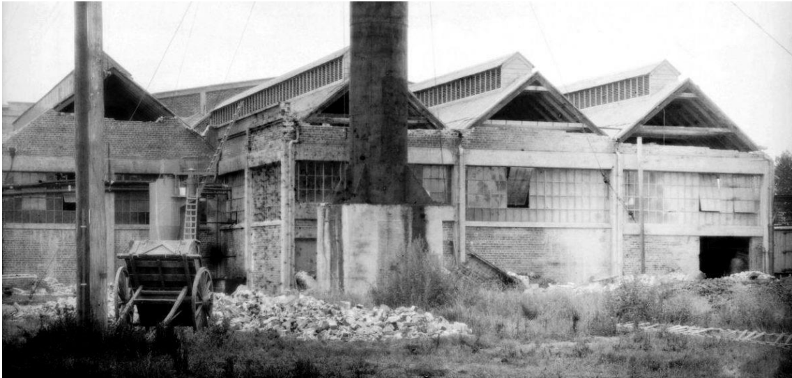
1931, Borthwick Freezing Works destroyed by the Quake
