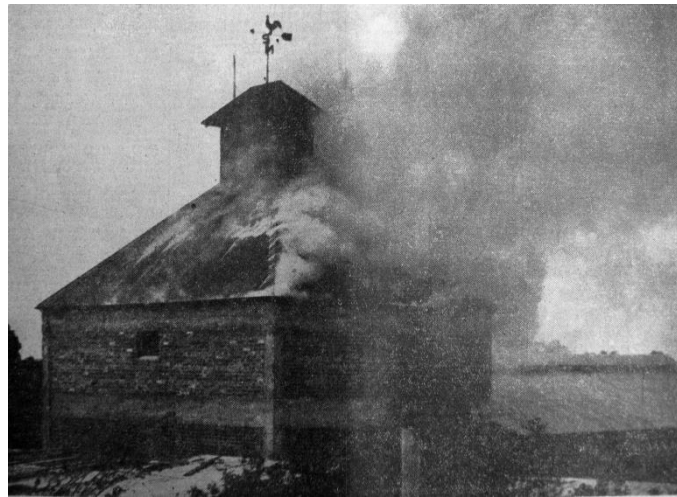
1939 January, Newbigin's Burton Brewery malt house on fire taken just prior to the brigade arriving. The brick and tin roof building supported by wooden beams was not in use at the time and its special ventilator in the roof enabled a terrific draft to circulate and fan the flames
