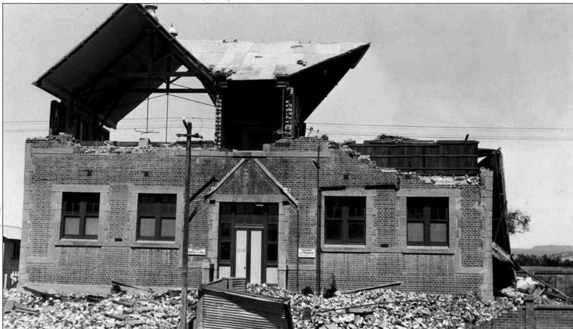
1931 February, The old Hastings Technical High School on Karamu Rd sth opposite the Gas Works demolished in the quake The sign on the left side of the door reads: School Dental Clinic; sign on the right side: Nurses, by Richard Savage
