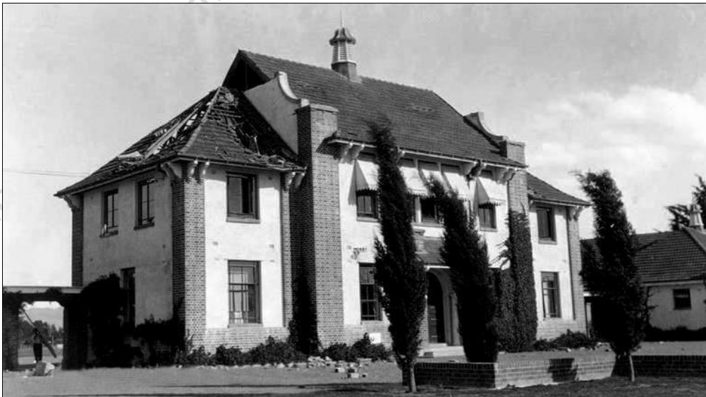
1931 February, Quake damage to roof
