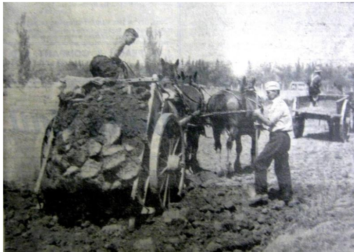
1939 February, The slow flood prevention work along the Ngararoro River at Pakowhai with horse & dump dray to build up the stopbanks
