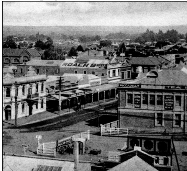
Roach Bros new premises
