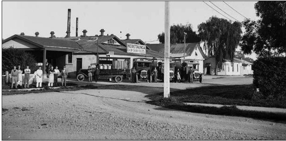
Heretaunga Co-operative Dairy Company Plunket St Stortford Lodge in 1932 taken from Stortford St
