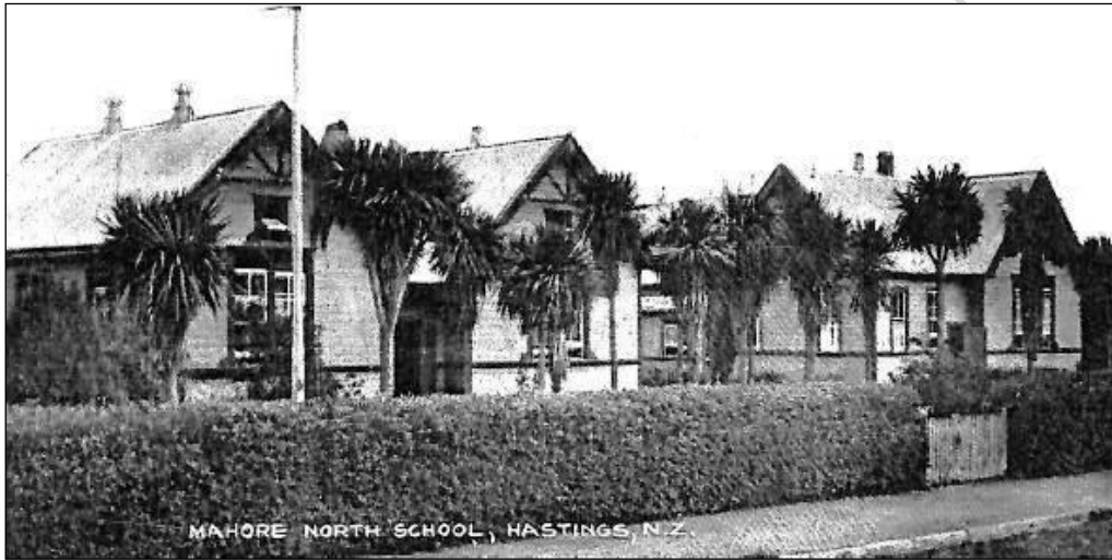
Later additions to the Mahora North school on Frederick St west
