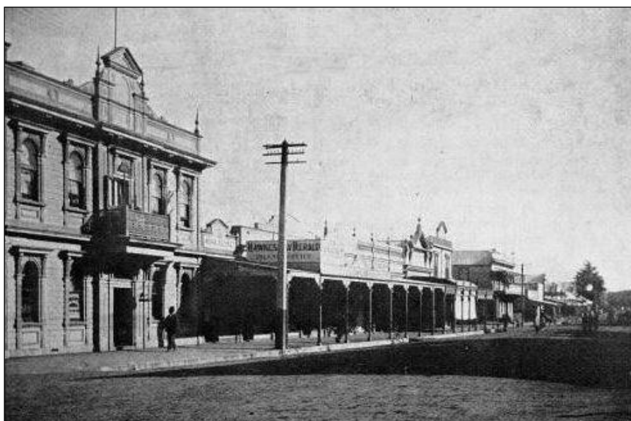
1902 July, Heretaunga St west from the railway, shows the Hastings Hotel left Hawke's Bay Herald and the Pacific Hotel with balcony further down
