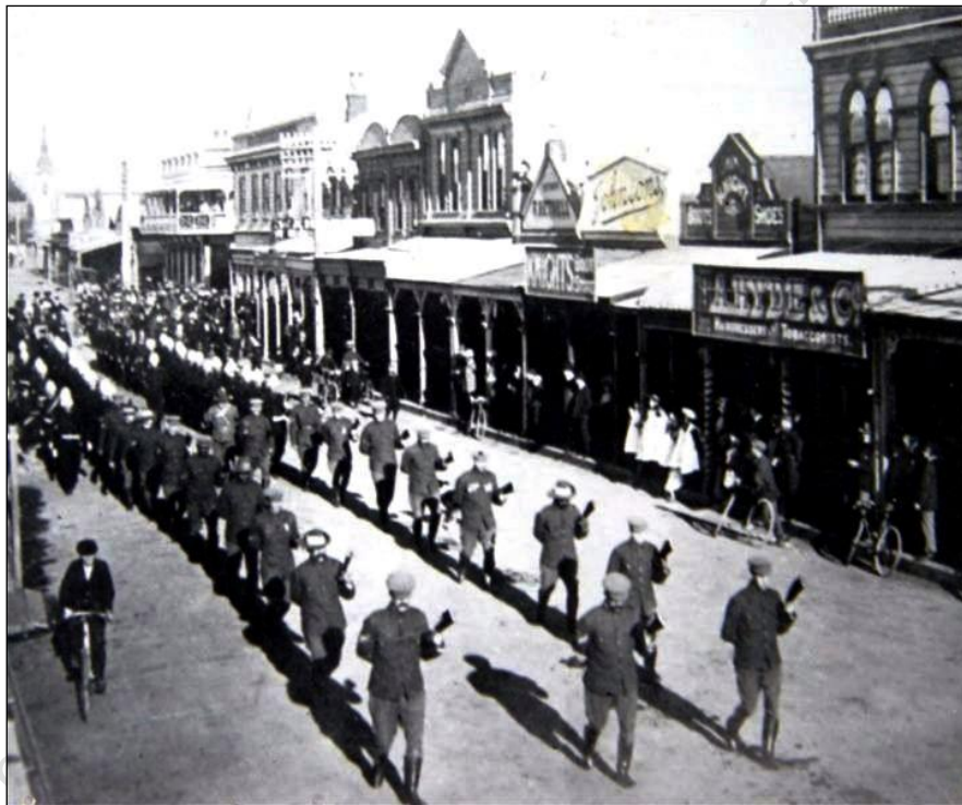
1906, Troops columns parade past the Grand Hotel construction site left on Heretaunga St east with arms reversed in respect for deceased PM Richard J. Seddon, with candy striped barber posts of A. Hyde & Co, with Albert & Carlton Club Hotels distant
