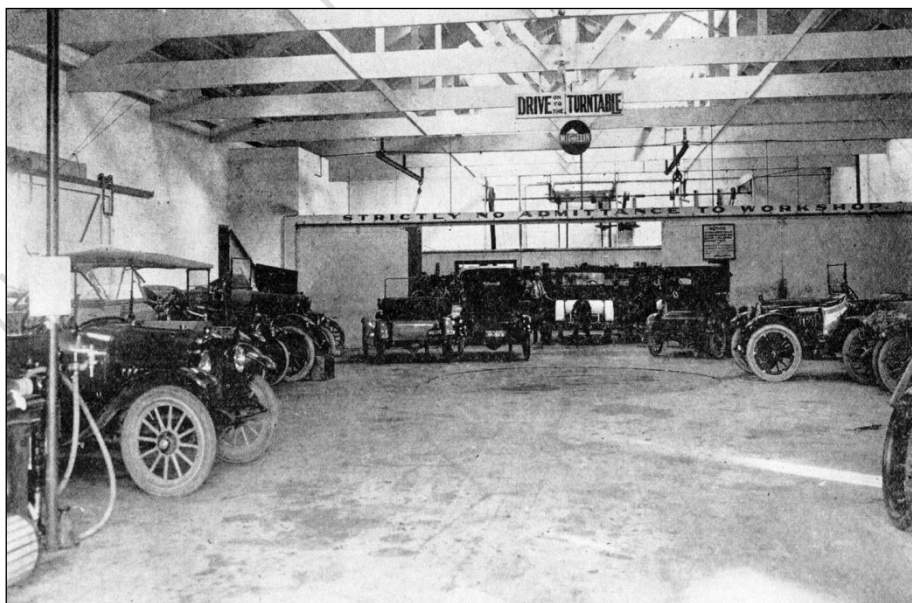
1915, Interior workshop of D. E. Davis & S. Boyd's new brick with concrete floor country garage 60 x 121 with a drive on turntable. In January 1915 Stanley Boyd's wife Ada died and the partnership of Davis & Boyd dissolved, David E. Davis continued on his accord
