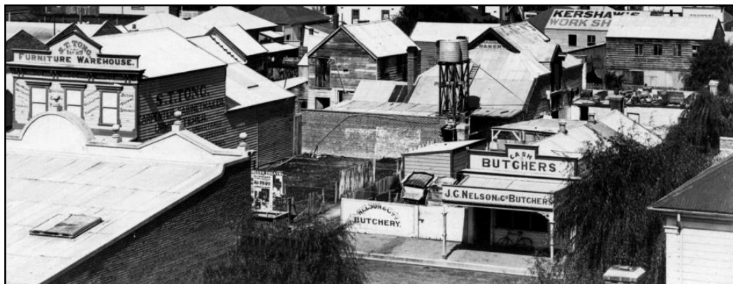
Looking east shows signage J. C. Nelson cash butchers at 105 Karamu Rd nth, S. T. Tong left and Warrens Bakery signage with two water tank towers behind and Kershaw's second work shop behind their Heretaunga St east store
