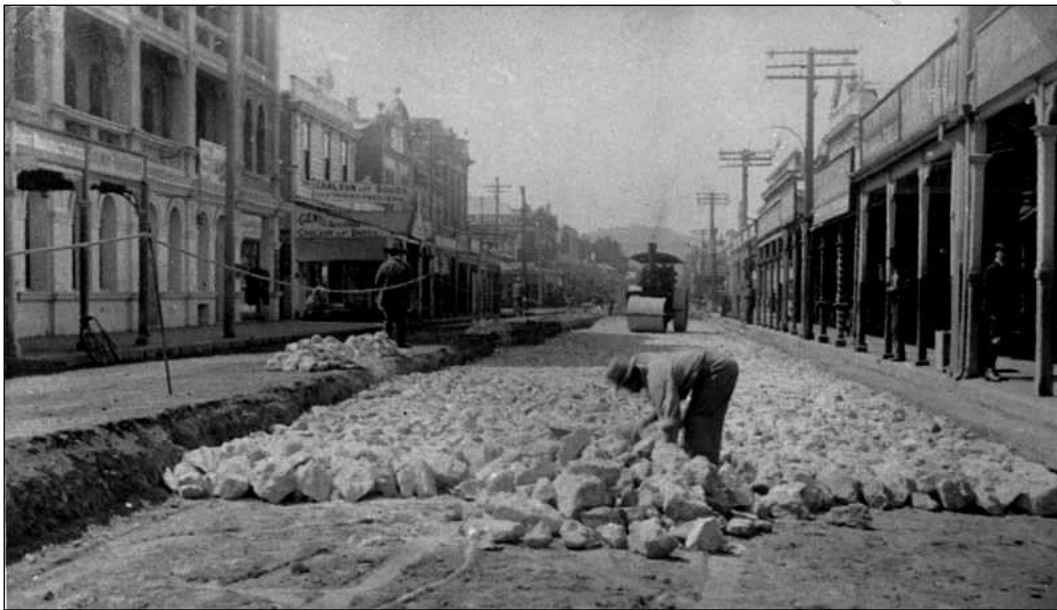
1914 August, Heretaunga St east road repairs outside the Grand Hotel using Shell Rock spalls possibly sourced from Fernhill, by Clapham
