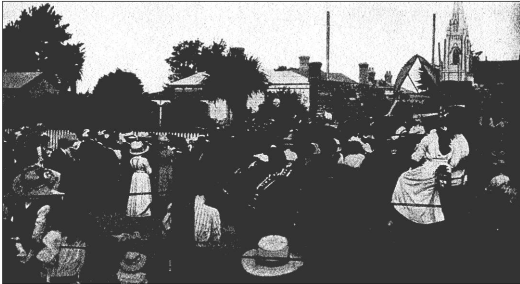
1912 February, Laying the foundation stone for the new Wesley Methodist Church in Hastings St sth. The Rev. G W. J Spence, president New Zealand Wesley Methodist Conference is addressing the audience. Mr James Garnett, Mayor, performed the ceremony of laying the stone. The pastor of the church is Rev. T. J. Wallis. Shows houses and the Catholic presbytery and church steeple on Heretaunga St east in background, by G. S. Clapham
