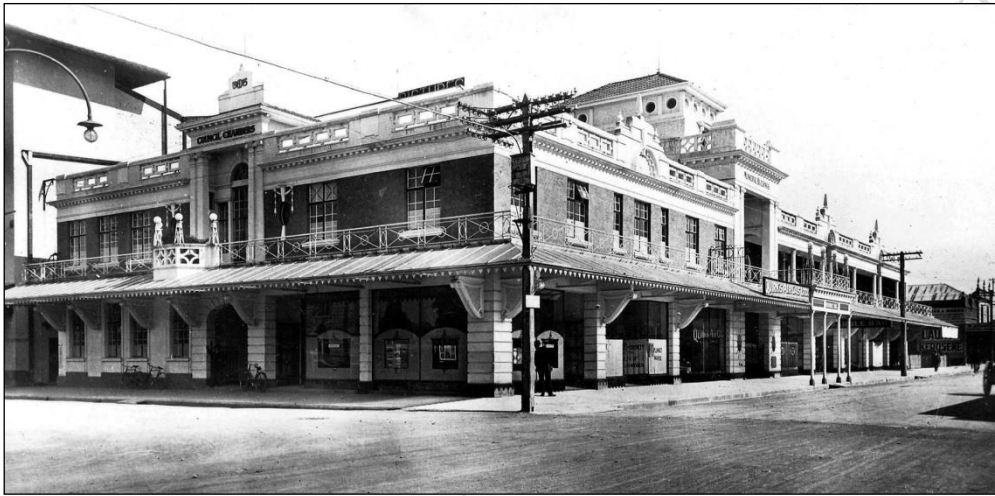
The Municipal Buildings Heretaunga St east, with signage for Laurel Kerosene distant
