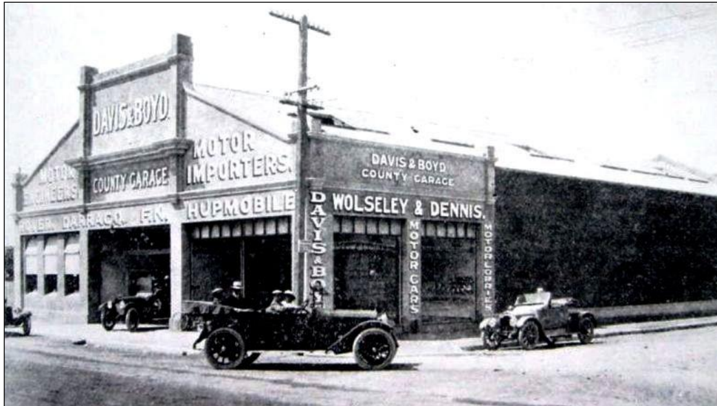
1915, D. E. Davis & S. Boyd's new brick with concrete floor Country Garage 60 x 121 on the corner of now Station St and Avenue Rd east opposite the Hastings Railway Station, where they installed their first bowser with Dalgety adjoining their new premises at the rear on Avenue Rd east
