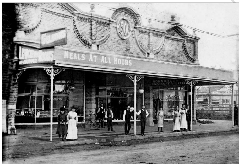
Three brick shops erected in 1906 for Mr W. A. Beecroft at 114 Karamu Rd nth opposite S. T. Tong, shows Gelhor's Luncheon Rooms and boarding house, poss later became The new Trocadero of the Hannah siblings till 1923. This building collapsed during the 1931 Earthquake
