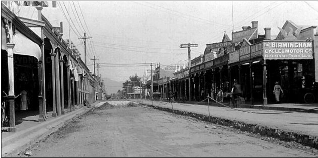
1914, Heretaunga St east road repairs now shows Birmingham Cycle & Motor Co, A. Simmonds, F. L. Bone, and Farrelly's boot and Millinery store, with possibly Farrelly's Bicycle Agents shop at 313 distant before the Catholic Church
