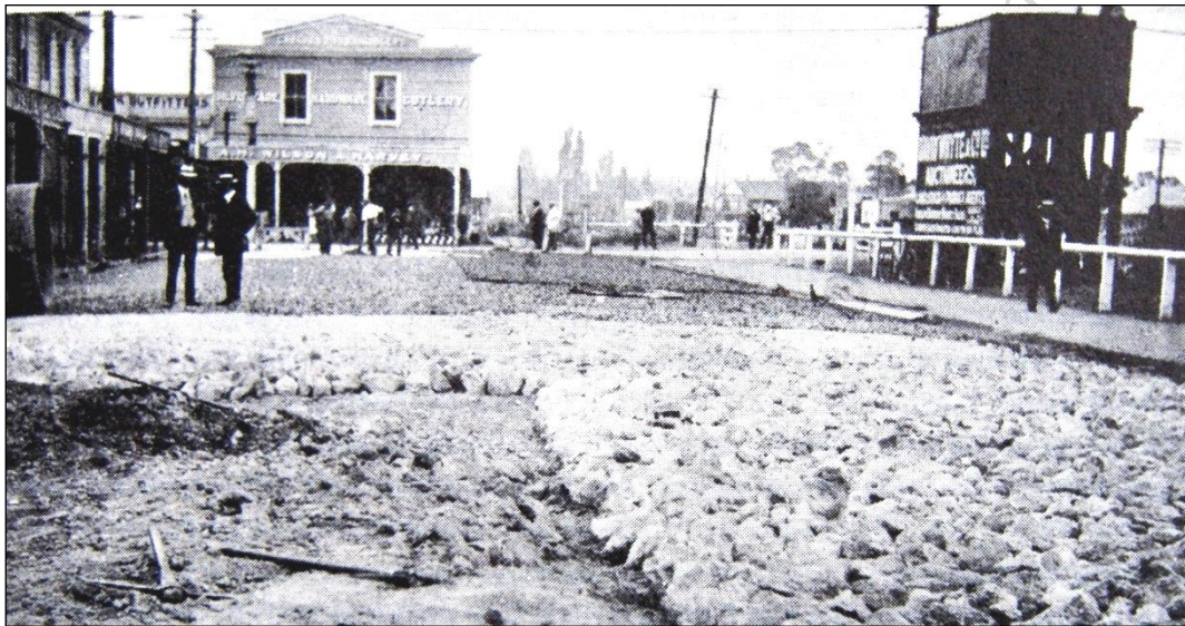
1914, Station St looking south, roadwork reconstruction using Shell Rock pass sourced from Fernhill - shows new A. H. Wilson & Harvey, Silverware, Hardware, Cutlery building before the Russell St extension after WW1 in 1920, R. Holts Timber yard has already gone
