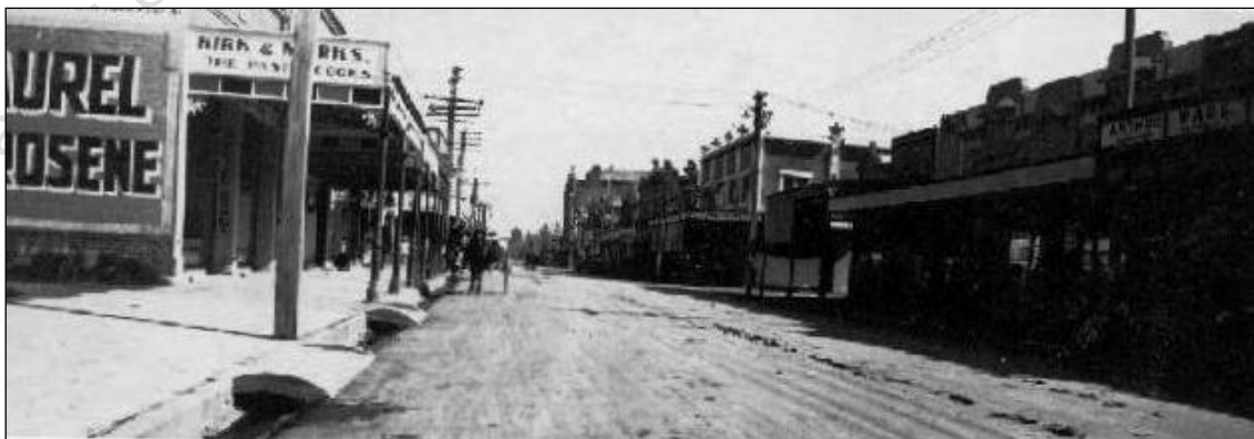
1917c, Heretaunga St east from near Salvation Army Citadel looking west with Laurel Kerosene signage and Kirk & Marks, with Arthur Wade plumbing at right 200 Heretaunga St east
