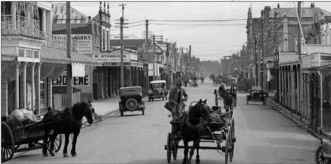
Heretaunga St east enlargement – the Municipal Buildings at right with signage for Laurel Kerosene, Kirk & Marks, W. Sturrock to Warren St, the Grand Hotel further left, by Sydney Charles Smith
