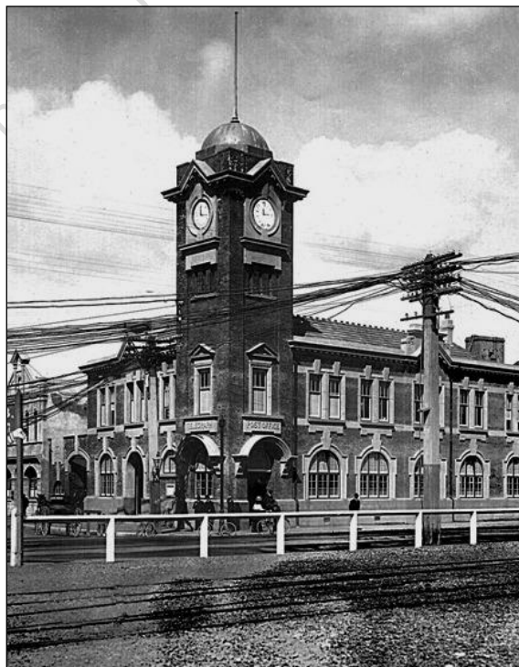
1912, from the Railway shows the new Post Office with telegraph pole heavy with cables going to the Telegraph office on Station St nth
