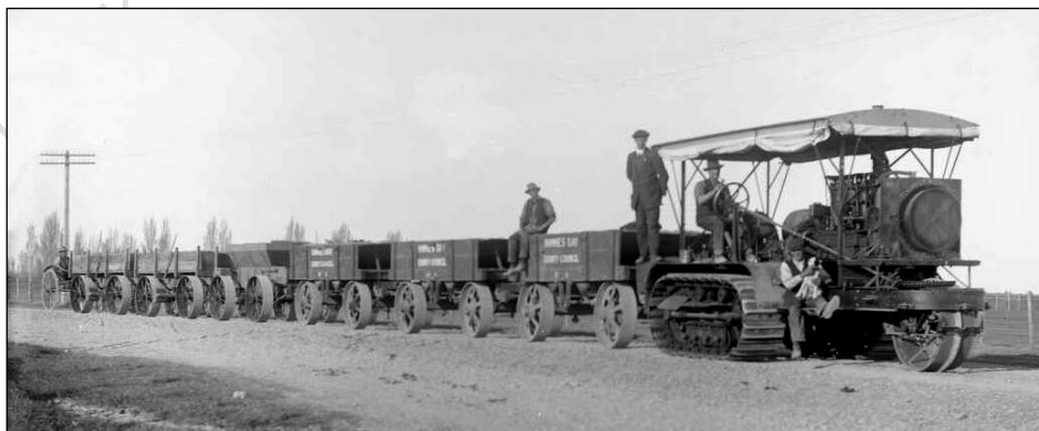
1911, Hawke's Bay County Council road construction team, bulldozer pulling wagons near Hastings, shows Tourist Motor Co Ltd, Agents, Hastings on the engine front
