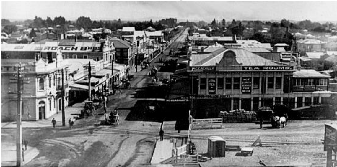
1912, Central Heretaunga St west shows the Piccadilly Tea Rooms of Miss England and McGlashan's signage after the 1907 Williams & Kettle fire with the removal of the tall fire bell tower to the new Fire Station on Market St. The tall old telegraph pole south side of railway track left with Hastings Hotel behind, Roach Brothers, the new brick Pacific Hotel and Princess Theatre in distant
