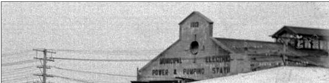
1912, The Edwardian Neo-Classic Municipal Electricity Power & Pumping Station building on Eastbourne St east built on the old Fire Station site behind the Borough Council Chambers, Electricity was now being generated by diesel oil engines and the Council had established a water reservoir on Mr Chambers site in Havelock and pumped reticulated artesian water through to most of the Hastings Borough which proved more satisfactory for fire fighting supply than the previously used drainage water, especially during the later 1931 earthquake, fluoride was added from 1954 at the new pump station on the corner of Havelock Rd and St. George's Rd. 1924 it was renamed the HB Electric Power Board and started supplying electricity in 1925
