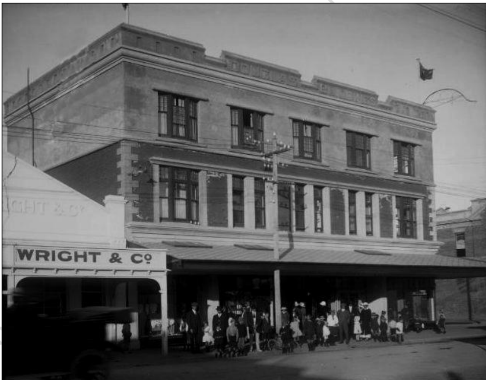
1920's, Heretaunga St west now shows the Harry Douglas building next to Phillips, Wright & Co builders, cabinet-makers at 411 – Joseph Phillip and H. W. Wright, with people waiting out front dressed in their finery late afternoon, NZ flags and an arch light pole, by Henry Norford Whitehead
