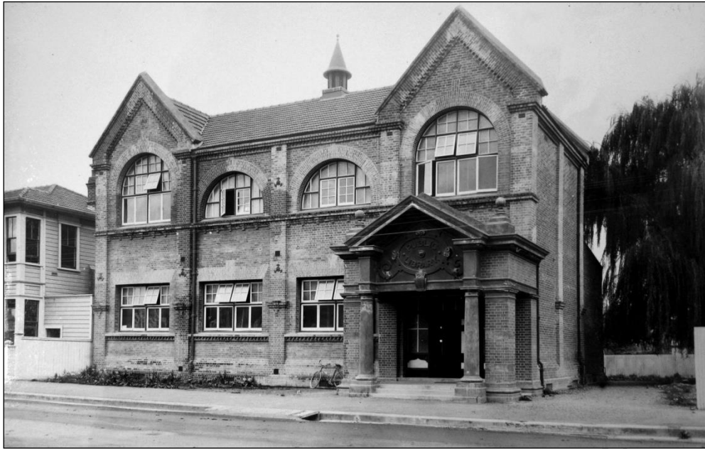
The Andrew Carnegie Hastings Public Library building in Market St sth constructed of brick in Queen Anne style designed by Napier architect Mr C. A. Vautier., on the ¼ acre section of James Boyle's, having frontage of 82½ft and a depth of 132ft and which the Borough Council had taken over for public use in October 1901. The old wooden Athenaeum was removed to the rear taken before driveway gates installed, the adjoining new wooden Hastings Club built 1906 designed by George Sollitt.
