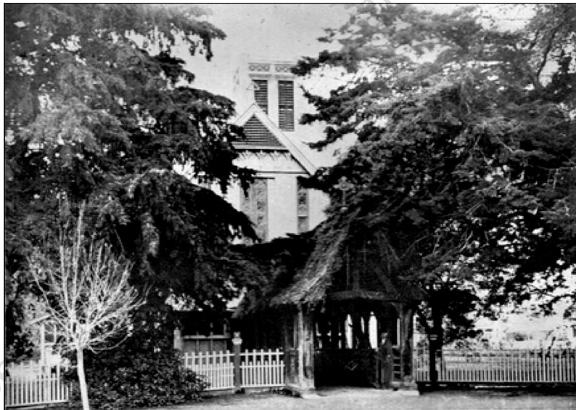
1930, St. Matthew's Church old rotted wooden lych-gate entrance King St sth with new concrete extension behind
