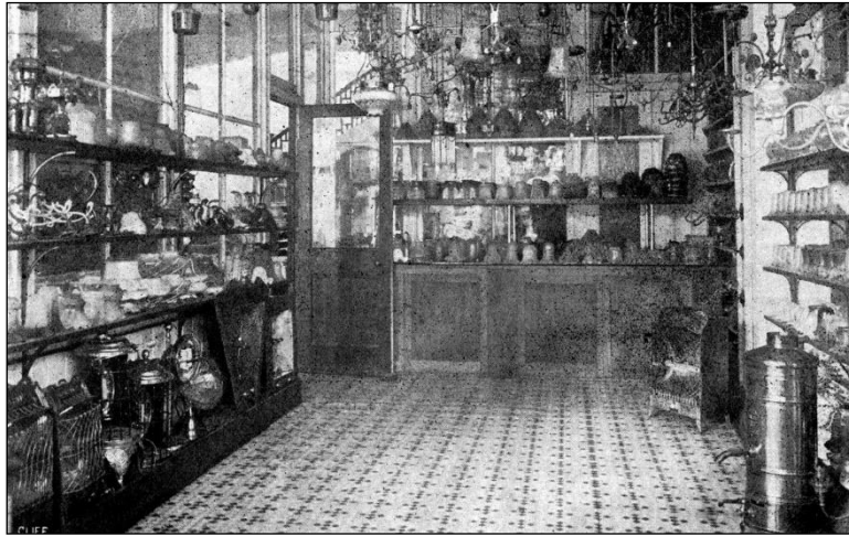
1917, Thomas Ritchie & Co, Electrical light showroom now Heretaunga St west by Roach's
