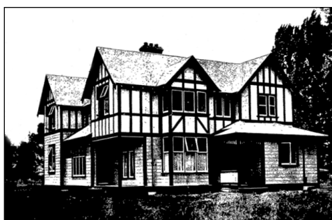
1909 June, Manager's House, to order of Mr Gaisford of Flaxmere, (Rush & James, Architects).
