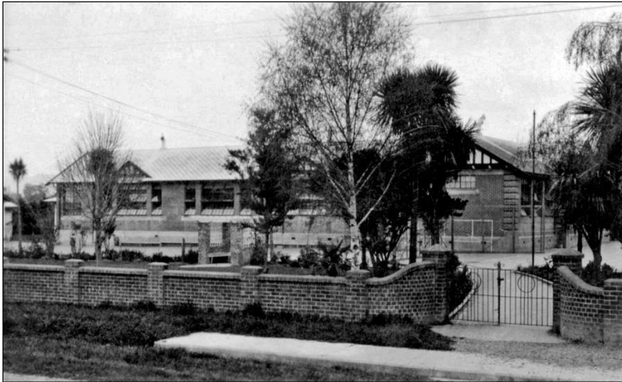
Parkvale School, shows entrance and end of new footpath
