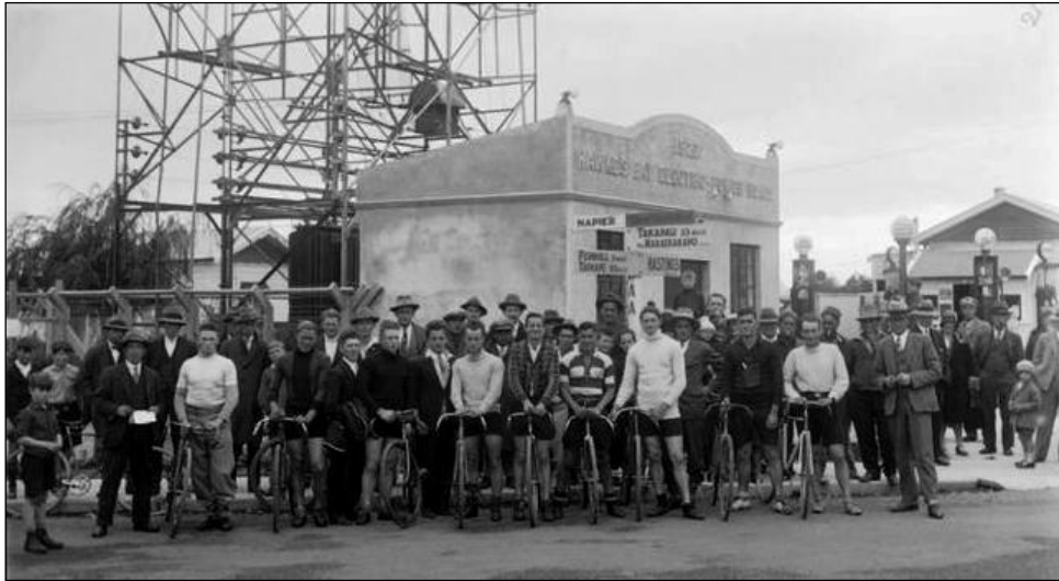
Cyclists at Stortford Lodge, Hawke's Bay Electric Power Board substation 1927 and the Premier Service Station Ltd bowsers, poss of D. G. Round
