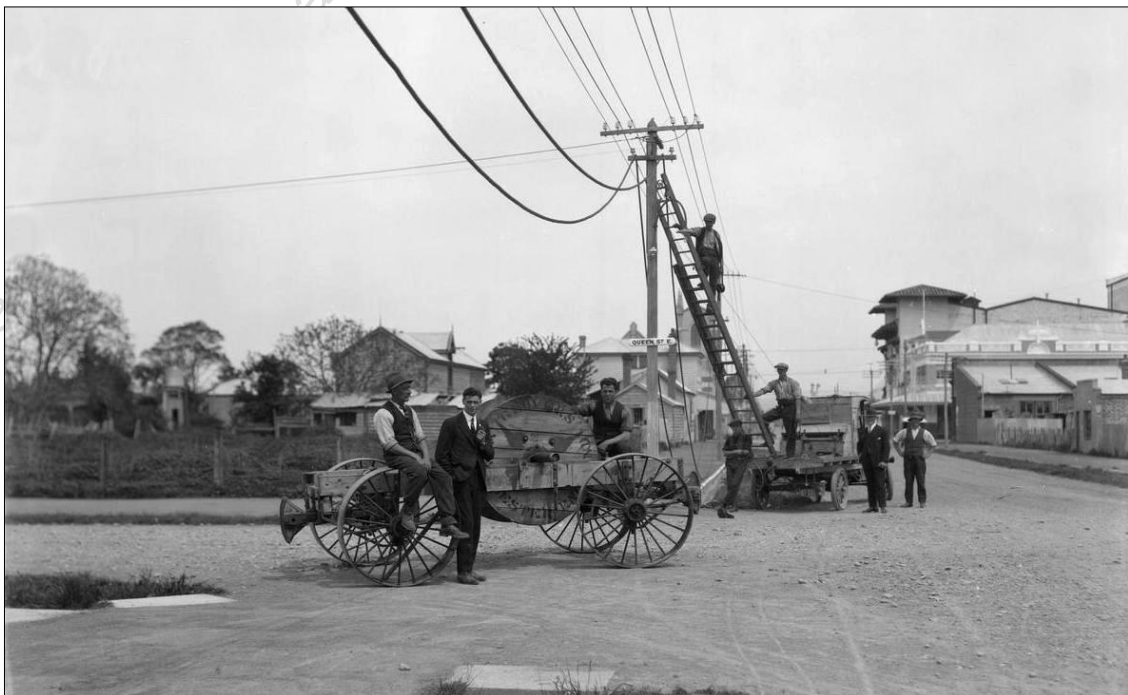
1920's, Workers installing electric power lines along Hastings St nth at the corner of Queen St east with Cullen's two story residence, store and bakery, the new Hastings Wesley Methodist Church behind left, the Hastings Municipal Theatre and right the Council Chambers on Hastings St right, a trailer supports a large wooden cable reel foreground, by Sorrell and son
