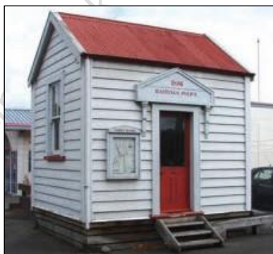
The small renovated historic Hastings Police station hut built 1879 - without its chimney, by Don Task
