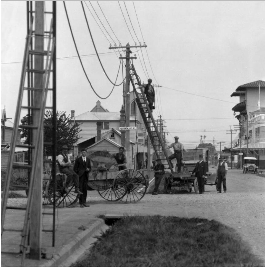
1920's, Workers installing electric power lines along Hastings St nth at the corner of Queen St east with Cullen's two story residence, store and bakery, the new Hastings Wesley Methodist Church behind left, the Hastings Municipal Theatre and right the Council Chambers on Hastings St right, a trailer supports a large wooden cable reel foreground, by Sorrell and son
