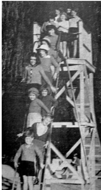
Children lining up to take a turn on the wooden slide at Cornwall Park during school holidays
