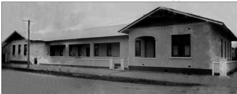
1927, Jesmond House, a private hotel at 311 Queen St west at the corner of Nelson St in Hastings. Proprietor J. H. Tate
