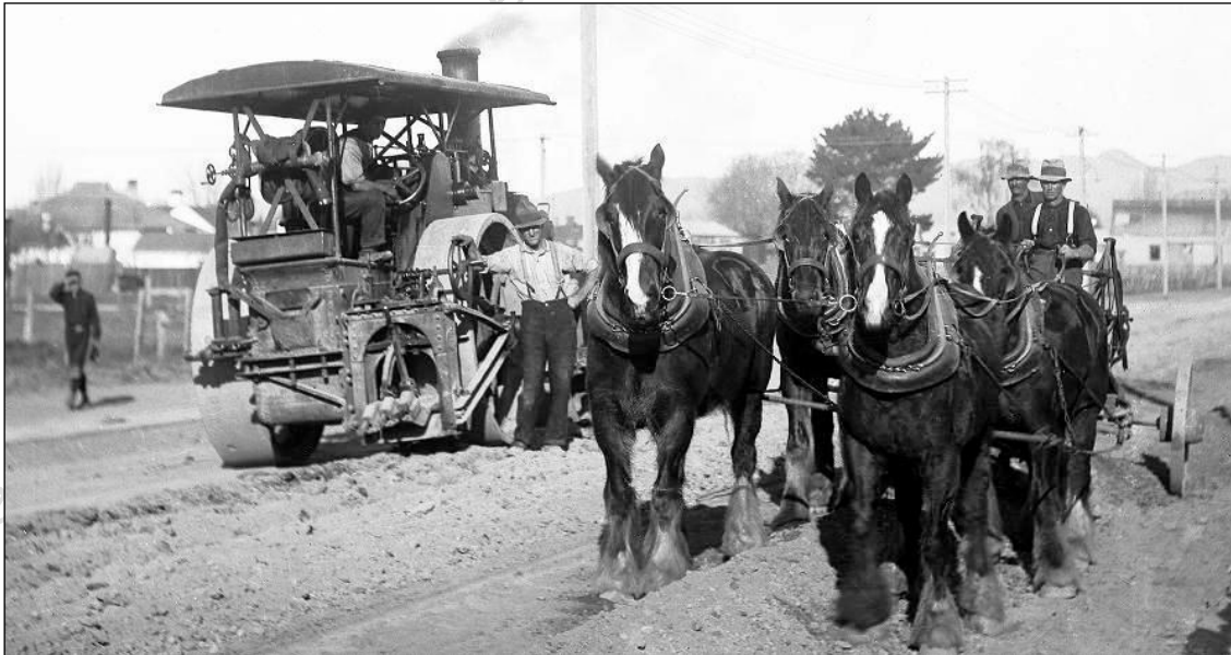
Heretaunga St west looking east with Tomoana Rd at left, road surface being renewed for the increasing demands of the motorcar, James Kitt and George Leslie driving the horse team grader with the steam roller and Council men standing behind, with schoolboy left with bag in gutter and child on footpath at right, Edward Matthews furniture manufacturer at 534 seen distant right at Charles St, horse & cart and man with shovel, excess soil used to fill in the Joll Rd, Quarry Rd pit for St. Leonard's Park, by Henry Norford Whitehead
