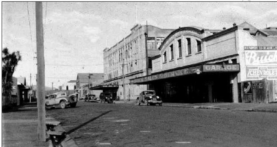
1930, Queen St west looking towards the Market St and the railway shows the newly rebuilt concrete H B Farmers Cooperative building with William's & Kettle across the road on Market St nth, and the Hawke's Bay Farmers Co operative Associations Buick Sales & Service garage forefront at 206 Queen St west built 1925, run by Bill Greer
