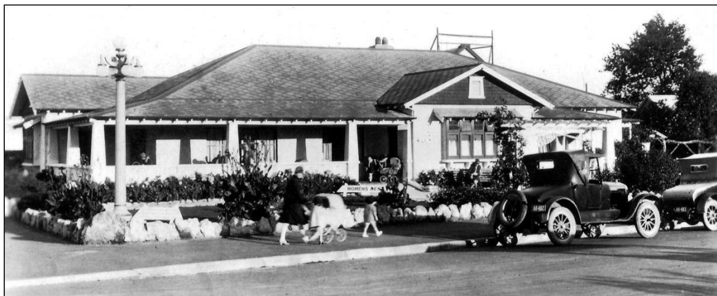
Woman's Rest Rooms corner of Eastbourne St east and Russell St with new street lighting
