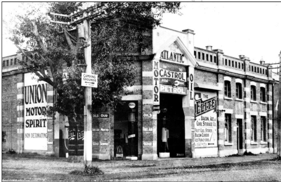
In 1926, Carl Vogtherr purchased the rest of Lowe Bros brick fronted cool store at Stortford Lodge corner of Maraekakaho Rd and Omaha Rd opposite the Hotel. The corner portion of the cool store was changed into a petrol station, son Ernie Vogtherr selling petrol brands such as Union, Plume, Big Tree, Texaco, Atlantic Castrol. Also shows signage for The Elite Bacon Ice and Cool Storage Co
