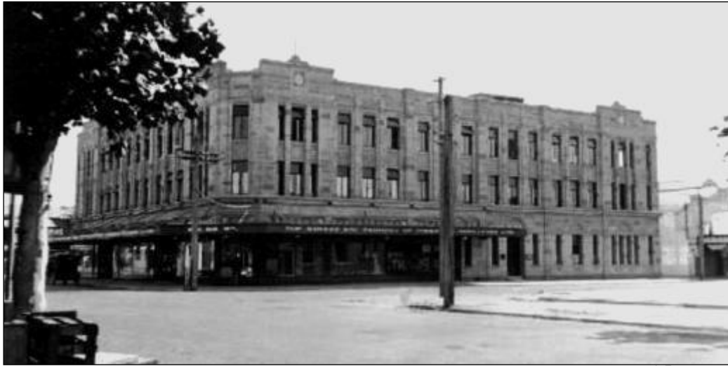
1930, The new rebuilt concrete H B Farmers Cooperative new building on Market St nth - the first building to have floating foundations and the Hawke's Bay Farmers Co operative Associations Buick Sales & Service garage at 206 Queen St west, designed by Edward [Edmund] Anscombe in 1929
