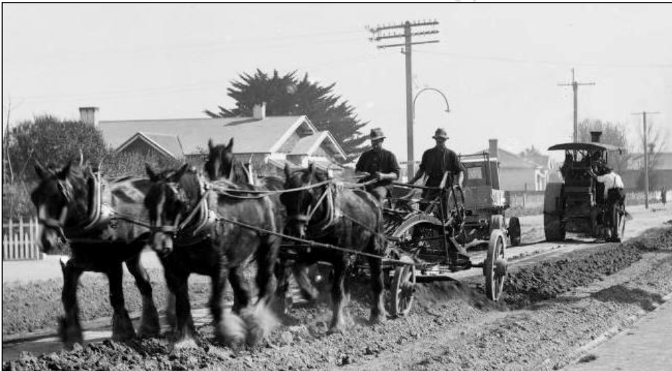
Heretaunga St west looking east, road surface being renewed for the increasing demands of the motorcar, with James Kitt and George Leslie driving the horse team grader with a steam roller and with schoolboy left, Tomoana Rd at left shows Smith, Scott & McHutchon, Blacksmiths, Wheelwrights & Coachbuilders at 111 Tomoana Rd, who later built the bodywork for the new Dennis fire engine for the Hastings Fire Board, side wall signage - Coach & Motor Body Builders, business partnership established after Charles Ferguson McHutchon had returned from WW1, shows schoolboy left, excess soil used to fill in the Joll Rd, old Quarry Rd pit for St. Leonard's Park, by Henry Norford Whitehead
