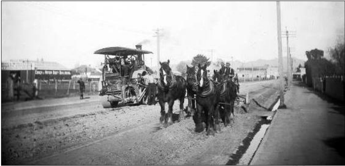
Heretaunga St west looking east, road surface being renewed for the increasing demands of the motorcar, with James Kitt and George Leslie driving the horse team grader with a steam roller and with schoolboy left, Tomoana Rd at left shows Smith, Scott & McHutchon, Blacksmiths, Wheelwrights & Coachbuilders at 111 Tomoana Rd, who later built the bodywork for the new Dennis fire engine for the Hastings Fire Board, side wall signage - Coach & Motor Body Builders, business partnership established after Charles Ferguson McHutchon had returned from WW1, shows schoolboy left, excess soil used to fill in the Joll Rd, old Quarry Rd pit for St. Leonard's Park, by Henry Norford Whitehead
