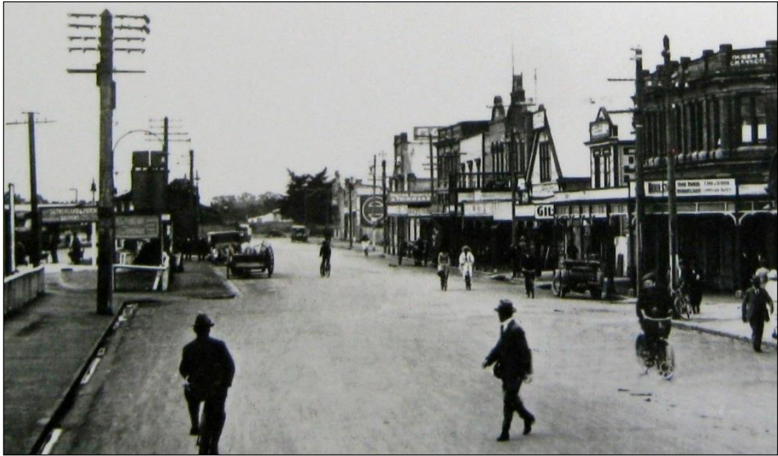
Early 1920's enlarged, looking north along renamed Russell St looking towards the Railway Station and St. Aubyn St distant with F. Cassin, Gill Brothers and McGlashan's old brick store on right further down, by Sydney Charles Smith
