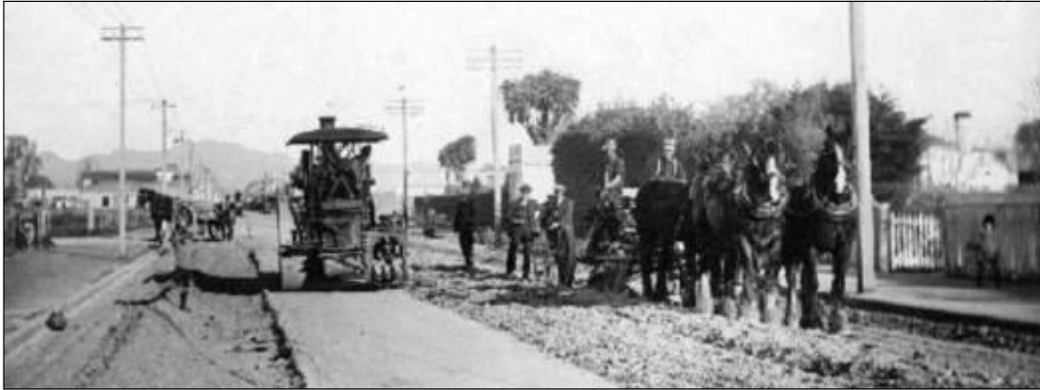
Heretaunga St west looking east with Tomoana Rd at left, road surface being renewed for the increasing demands of the motorcar, James Kitt and George Leslie driving the horse team grader with the steam roller and Council men standing behind, with schoolboy left with bag in gutter and child on footpath at right, Edward Matthews furniture manufacturer at 534 seen distant right at Charles St, horse & cart and man with shovel, excess soil used to fill in the Joll Rd, Quarry Rd pit for St. Leonard's Park, by Henry Norford Whitehead
