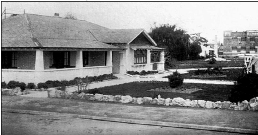
Mother's Rest Rooms built August 1921, corner of Eastbourne St east and Russell St – on a section given by Mrs J. Garnett in 1921 on condition of open space, shows the WW1 Cenotaph and de Pelichet, McLeod & Co building. Mrs Hannah Garnett nee Wilson died May 1942 at Hastings aged 85 the widow of late James William Garnett.
