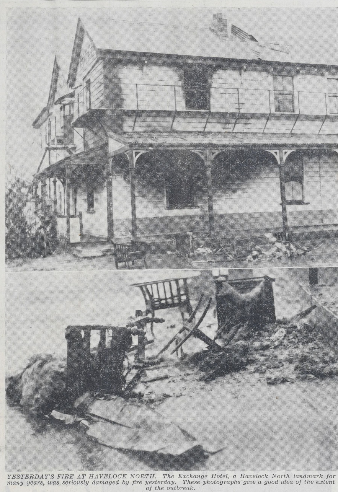
YESTERDAY'S FIRE AT HAVELOCK NORTH.—The Exchange Hotel, a Havelock North landmark for many years, was seriously damaged by fire yesterday. These photographs give a good idea of the extent of the outbreak.
