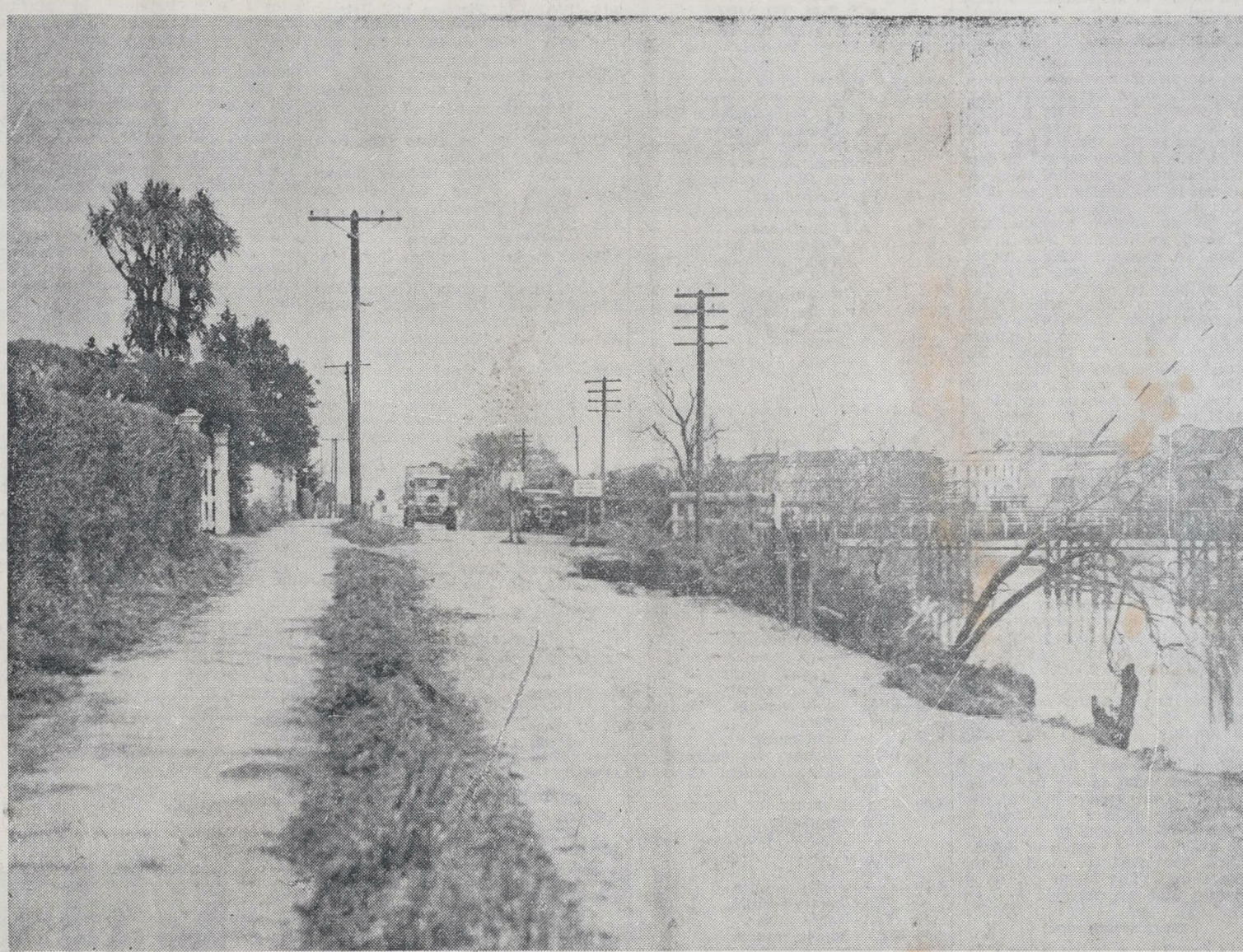
FLOOD DAMAGE AT GISBORNE.—A photograph showing the serious damage caused by the heavy rain and flooding of the Waimata River, Gisborne.
