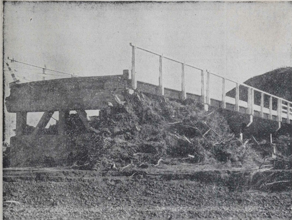
THIS WAS ONCE A BRIDGE. —The approach is all that is left of the main traffic bridge near the mouth of the Esk River.
