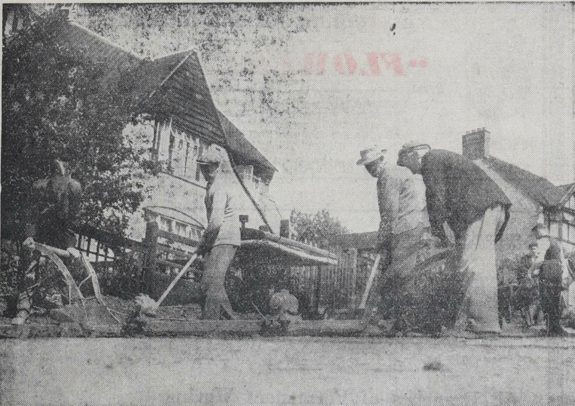
WHERE STEAMROLLERS FEAR TO TREAD.—In England, road vibrators are now used on gradients too steep for steamrollers.
