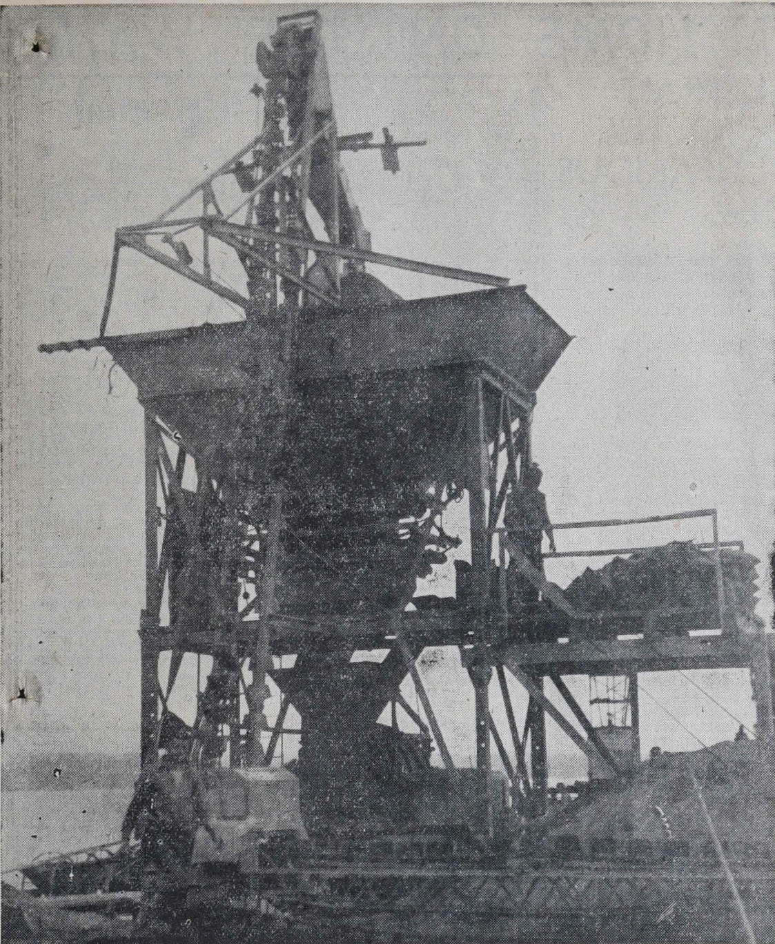
BREAKWATER EXTENSION WORK.—The great combination concrete-mixer at work on No. 1 wharf.
