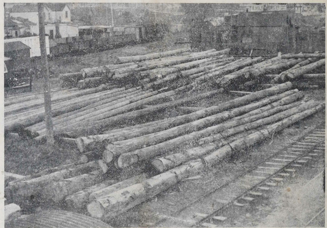
FOR EAST COAST RAILWAY CONSTRUCTION.—Bignum piles from the Dannevirke district in the Napier railway yards. Some of the logs are over 80ft. in length.
