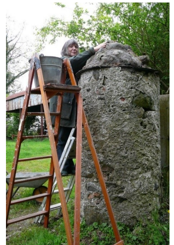
Figure 1 Clare Gulliver making repairs to a Thompson Leitrim farm gate post. PHOTO - CLARE GULLIVER
