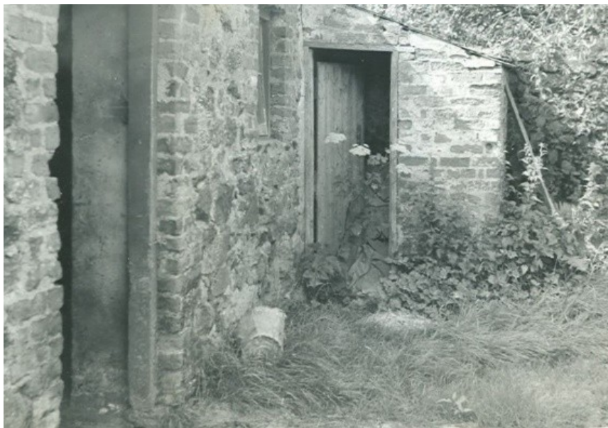
The old Leitrim Villa 'privy'
