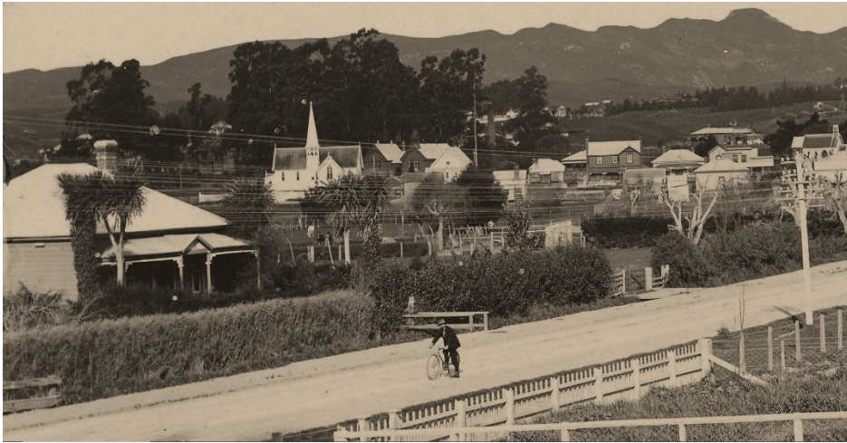
Figure 3 The first Thompson house that became familiar to everyone after crossing the bridge despite its growing decrepitude ...
