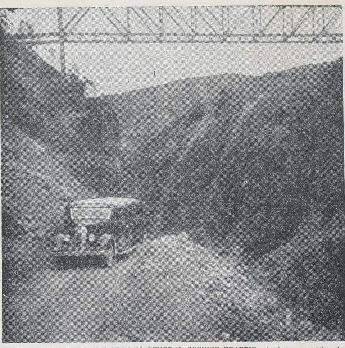
NAPIER-WAIROA ROAD NOW OPEN TO GENERAL SERVICE TRAFFIC.—A photograph taken by the "Daily Mail" cameraman of the service car negotiating one of the sharp bends on the narrow road at the point where the railway passes over the highway.
