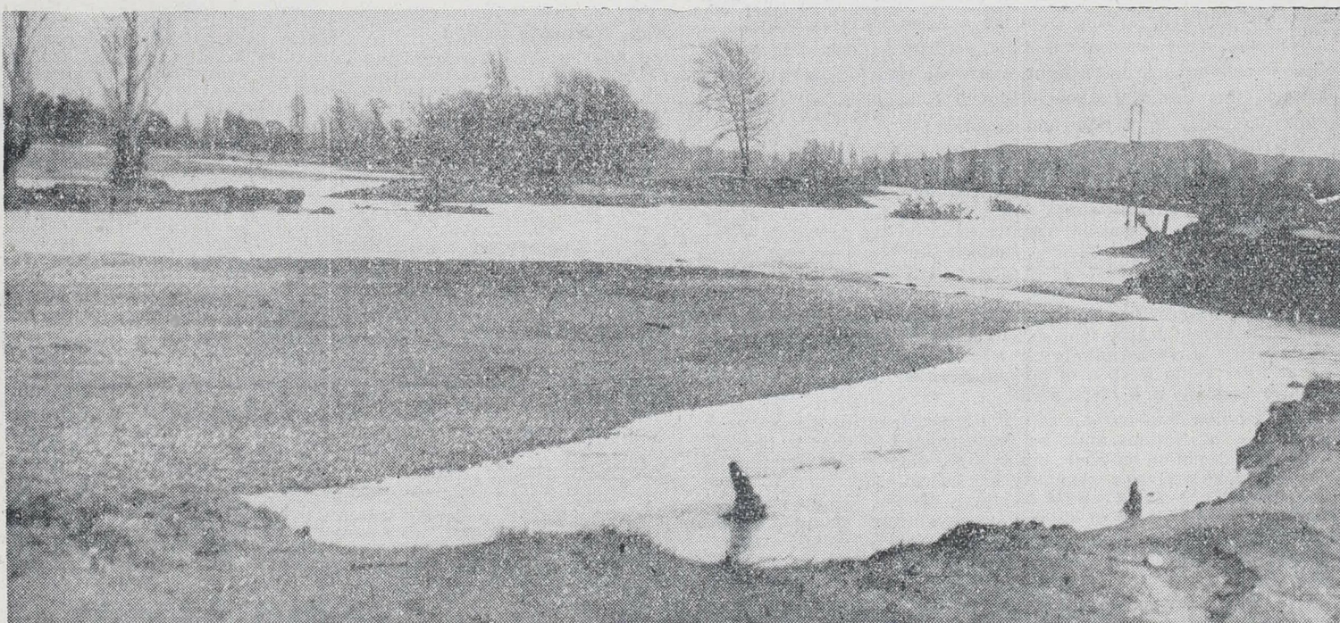
LOOKING UP THE NGARURORO RIVER NEAR CHESTERHOPE.—On the right can be seen the new cut which has straightened the river's course. The old bed was on the left. The last flood completed this change.
