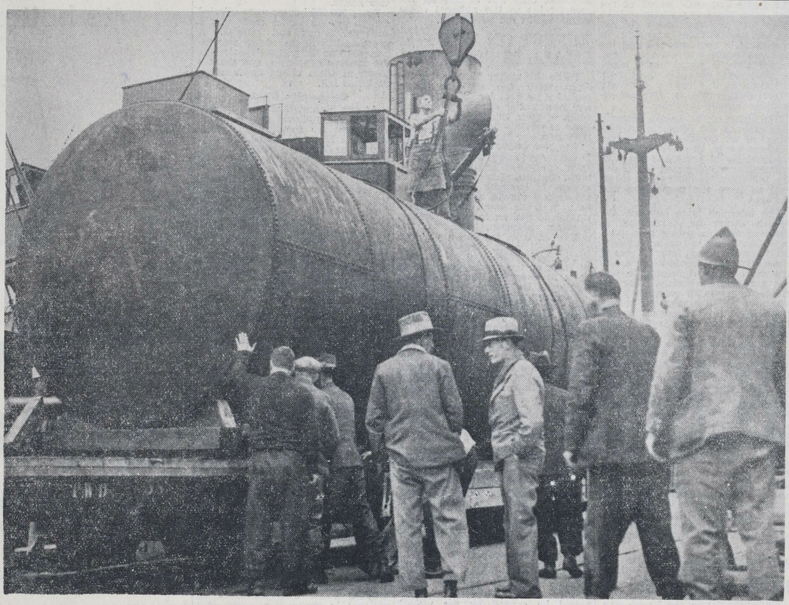
SEARCH FOR OIL NEAR GISBORNE.—A ten thousand gallon tank being unloaded at Gisborne wharf. It will be used for storing oil for the Diesel engines used in the boring plant.
