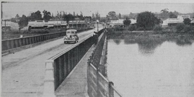
THE BUSINESS CENTER IN THE FAR NORTH OF THE PROVINCE.—A general view taken by the "Daily Mail" viaduct in the main road connecting North Otago with Waikato.
