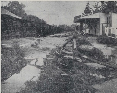
WRECKAGE AT THE ESK VALLEY RAILWAY STATION
