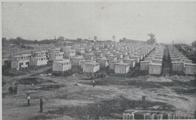
SOCIAL REFORM IN PORTUGAL. —Rows of houses built by the Portuguese Government to replace slum dwellings near Lisbon.
