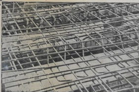
NEW NAPIER WHARF.—The intricate steel framework is now being reconstructed.
