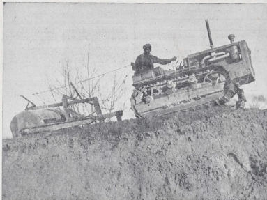
THE NEW WAY.—A two-gang mechanical scarp at work on the stonybank opposite Wahiata.
