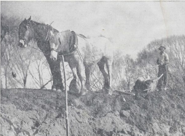
THE OLD WAY.—A horse-driven one-gang scarp on the 370-acre bank at Wahiata.
