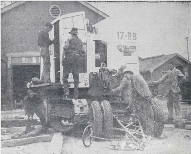
RIVERS BOARD'S NEW EXCAVATOR—A new excavator by Iny selected at Napier for the Hawke's Bay Rivers Board.
